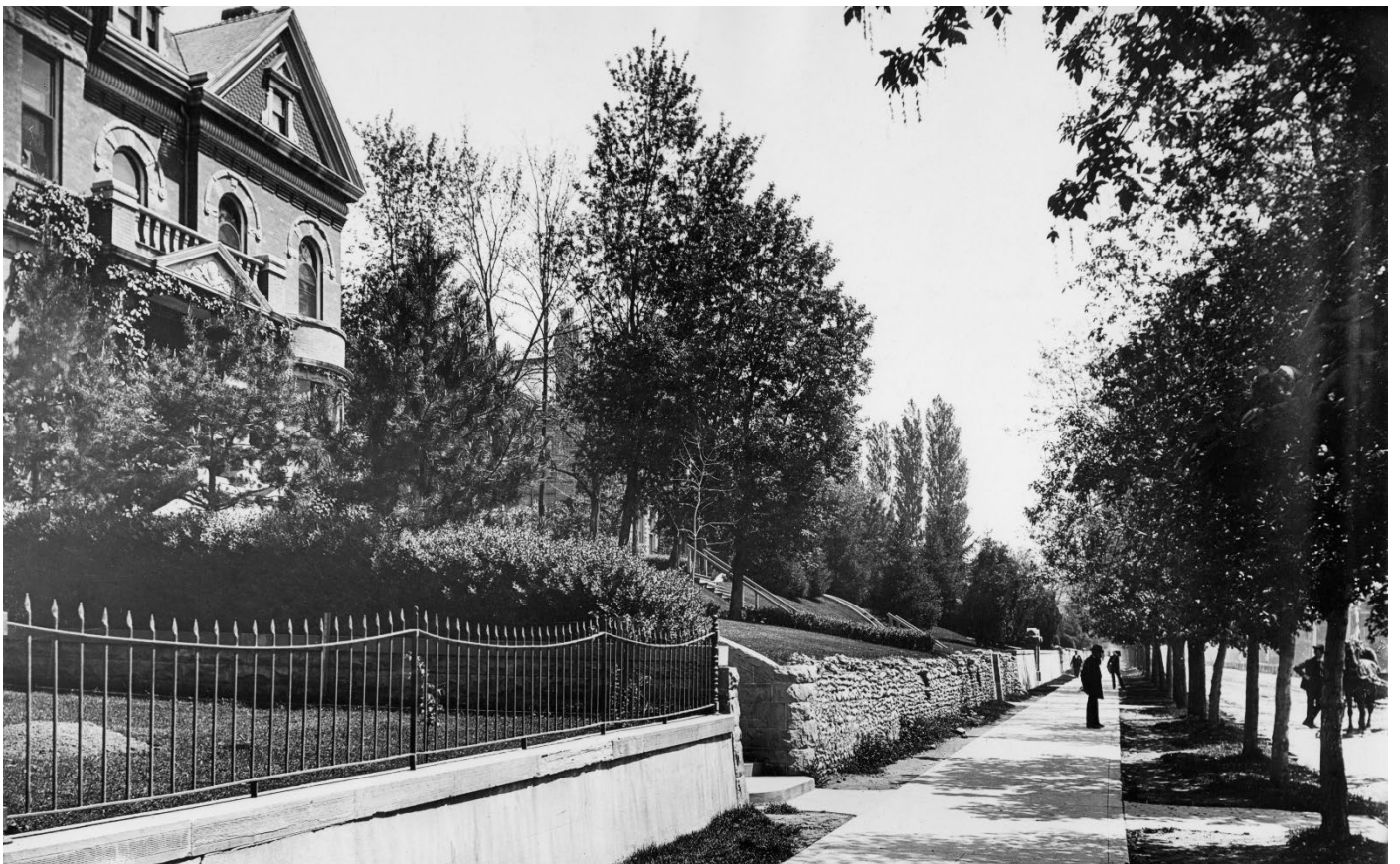
Elks Building Site – c.1910-1912
