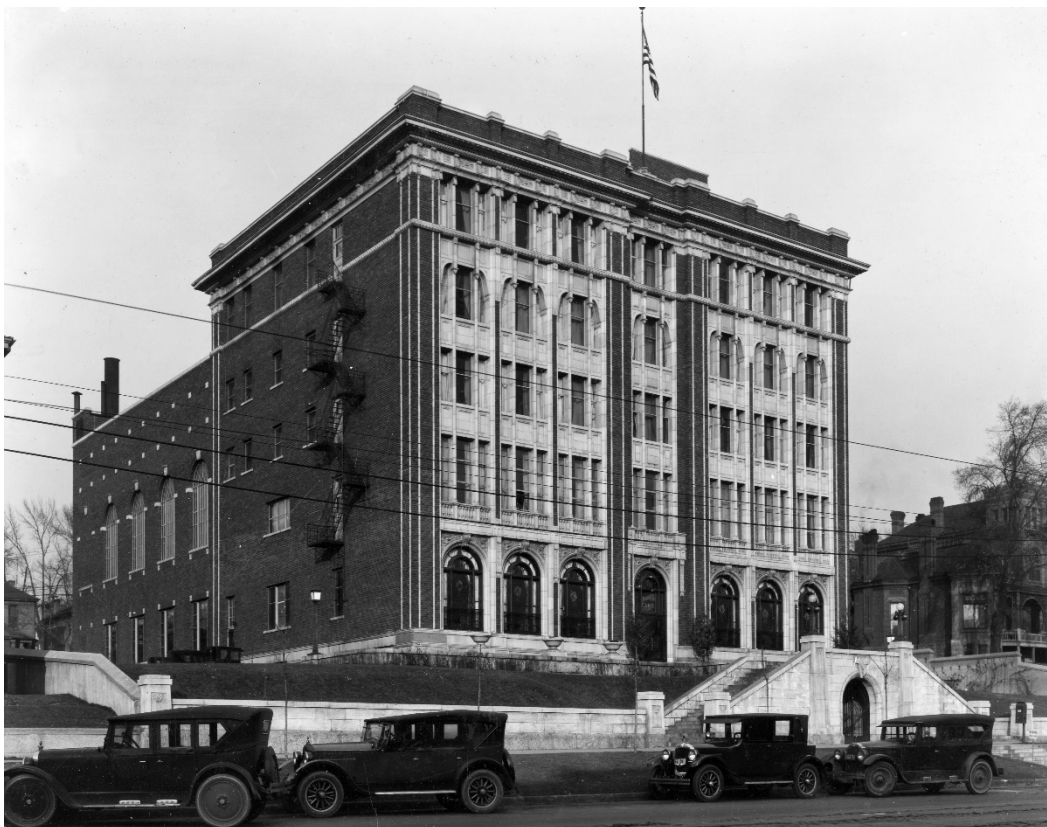
Elks Building – 31 December 1925
