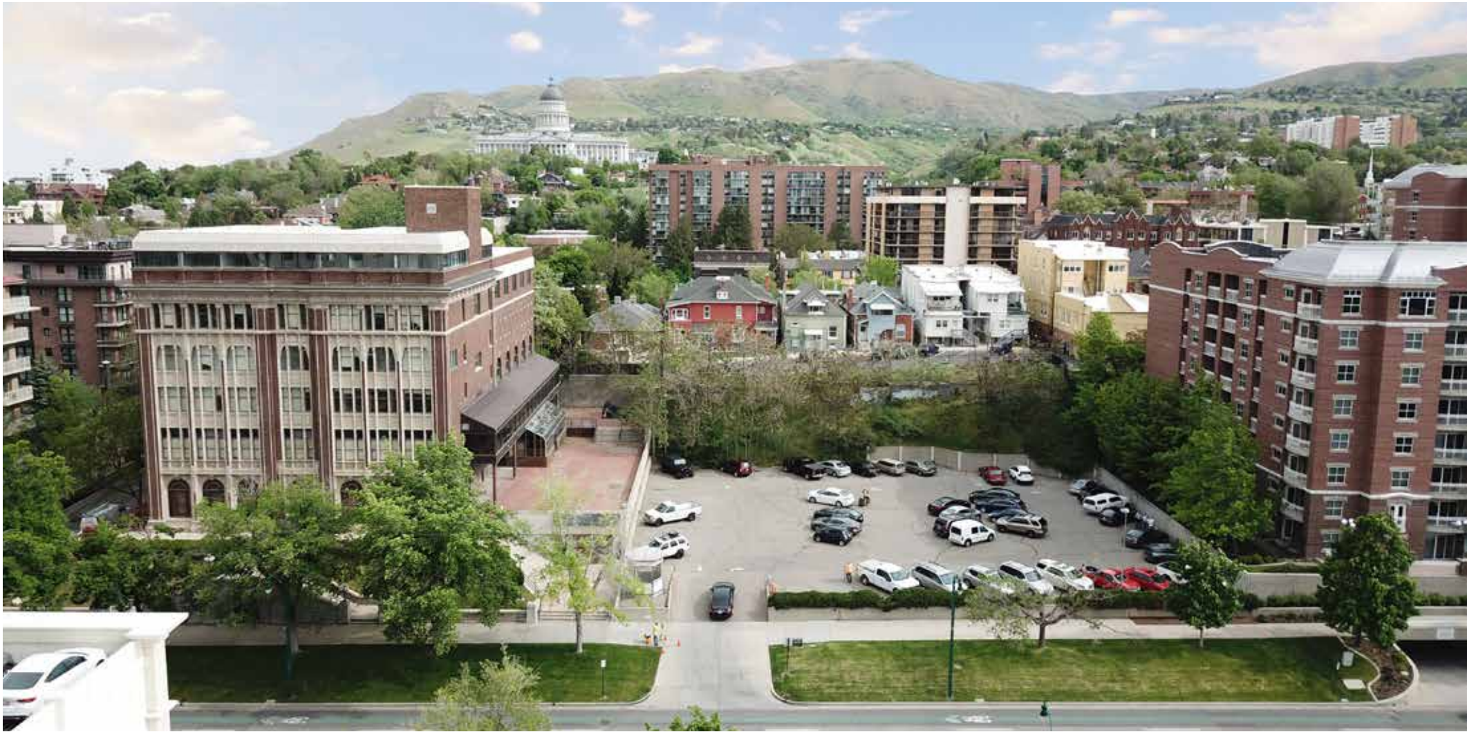
Existing Site Condition
