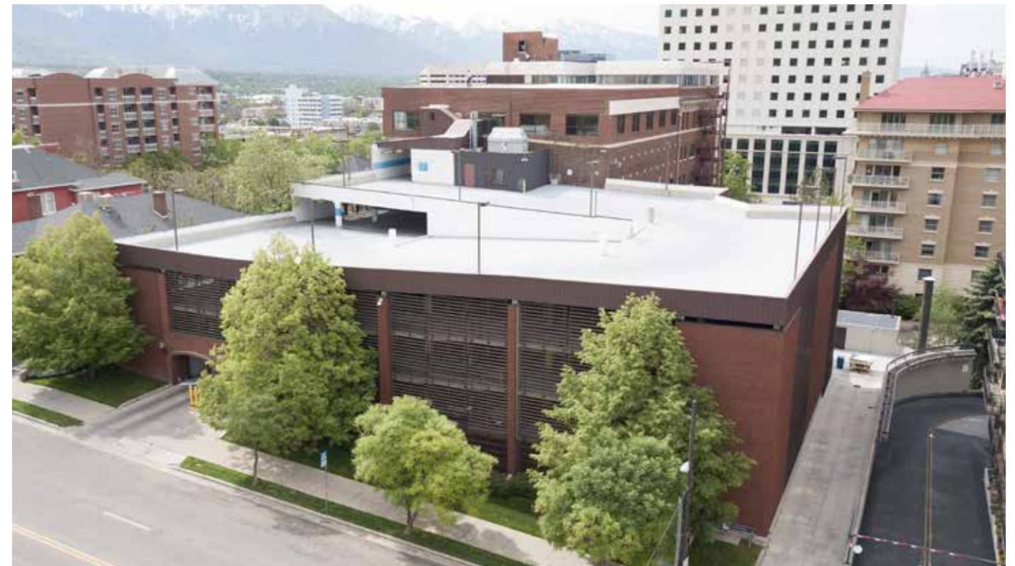
Existing Site Photos
