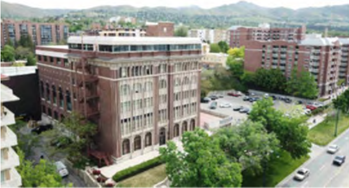
Existing Rooftop Addition
