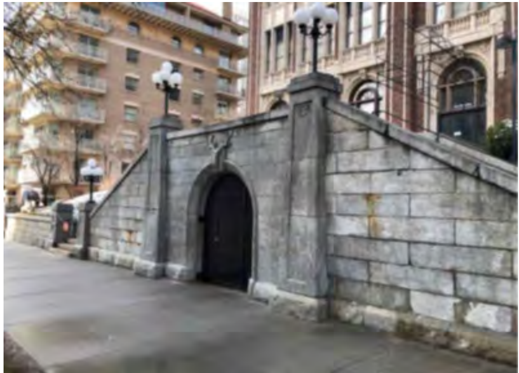
Current condition of building entry.
