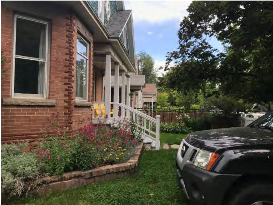
Facing north, alignment of front façades. The front façade of the proposed residence would be in alignment with the property to the north – the residence in the foreground with red brick.
