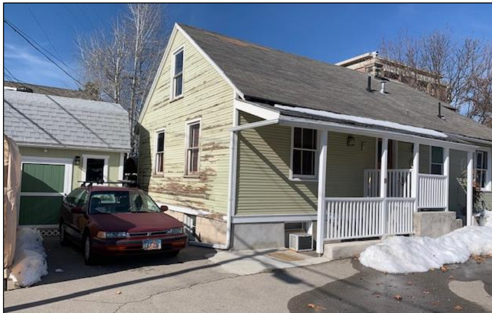
Photo of East and South Elevations
