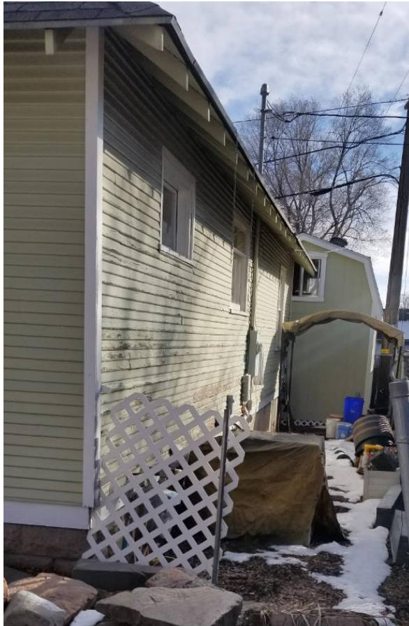
Photo of West Elevation
