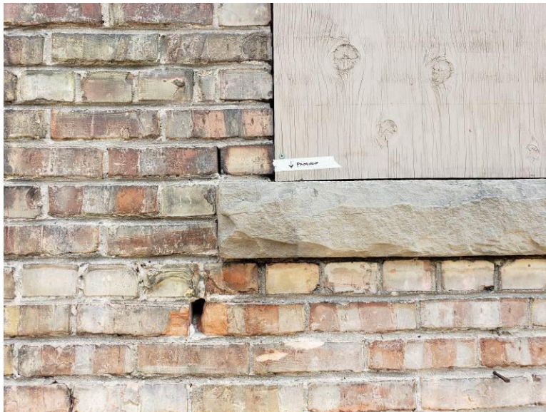
The location of the Prosoco test application, approximately two feet square to the lower left of the window on the west facade. The photo was taken after 35 days of drying. It has slightly darkened the stone window sill. The alteration of the brick is less apparent to the naked eye. The masonry will also be gently cleaned as a part of this project.
