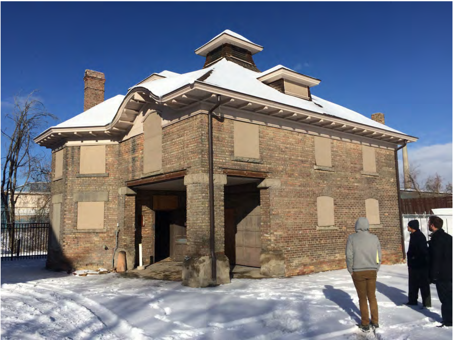
IMAGE 9: current photo of SE corner with carriage entrance portico, pre earthquake
