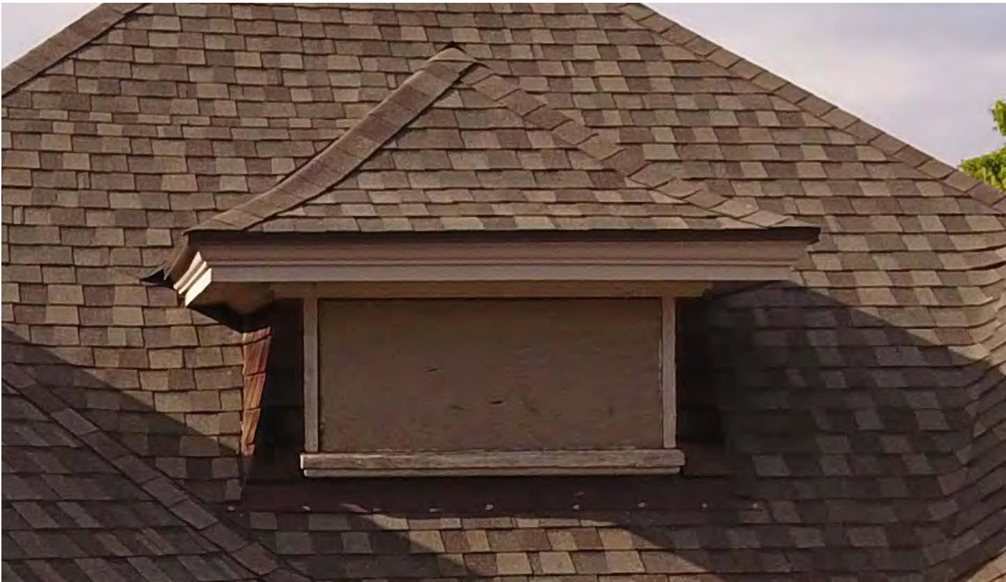
IMAGE 15: current photo of south dormer proposed to have its glazing replaced with louvers, post earthquake
