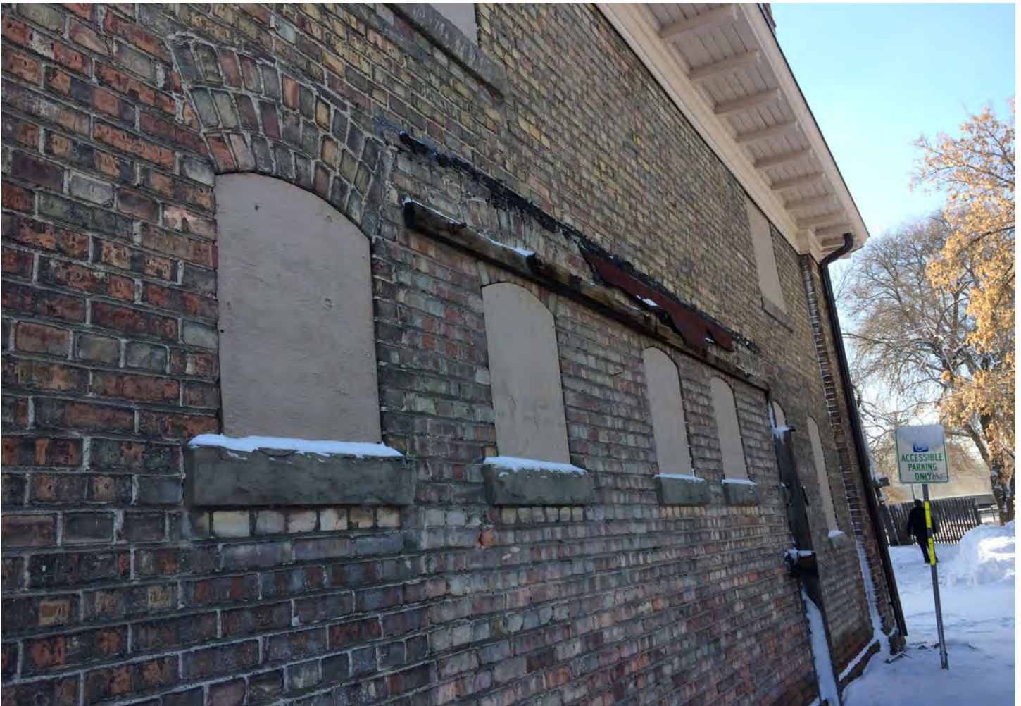
IMAGE 13: current photo of west facade, pre earthquake
