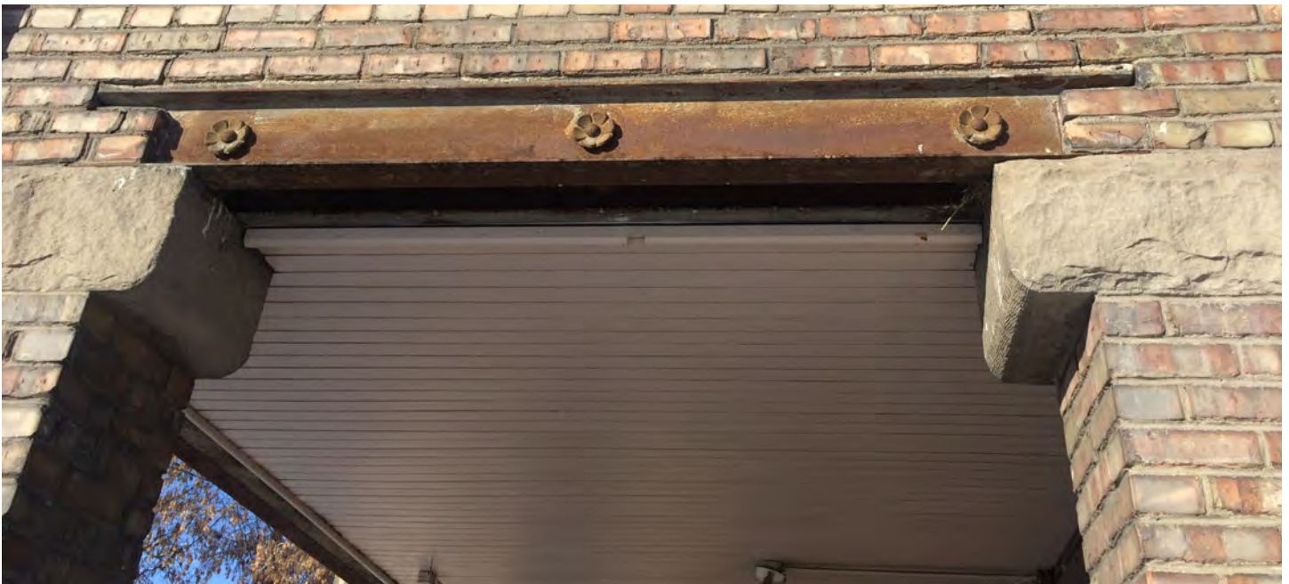
IMAGE 10: closeup photo of east carriage entrance portico, where storefront will be located, pre earthquake
