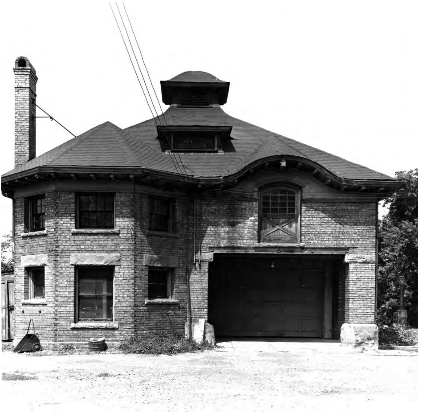
IMAGE 1: historic photo of south facade
