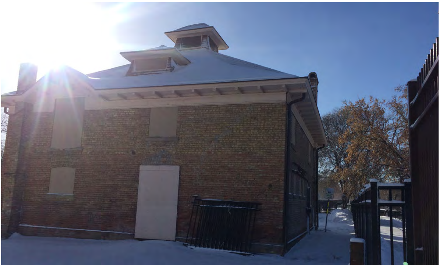
IMAGE 12: current photo of north facade, pre earthquake
