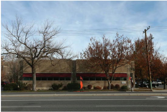
404 N. 300 W. BUILDING ON SOUTH END OF BLOCK
