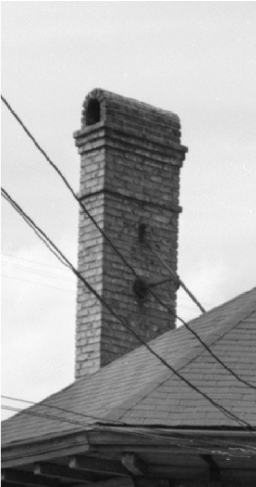
IMAGE 6: historic photo of south chimney
