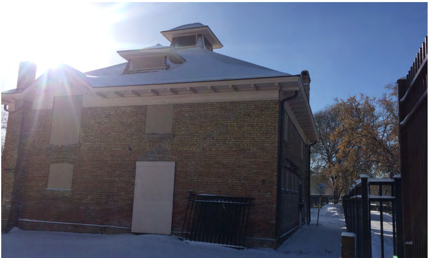
IMAGE 12: current photo of north facade, pre earthquake
