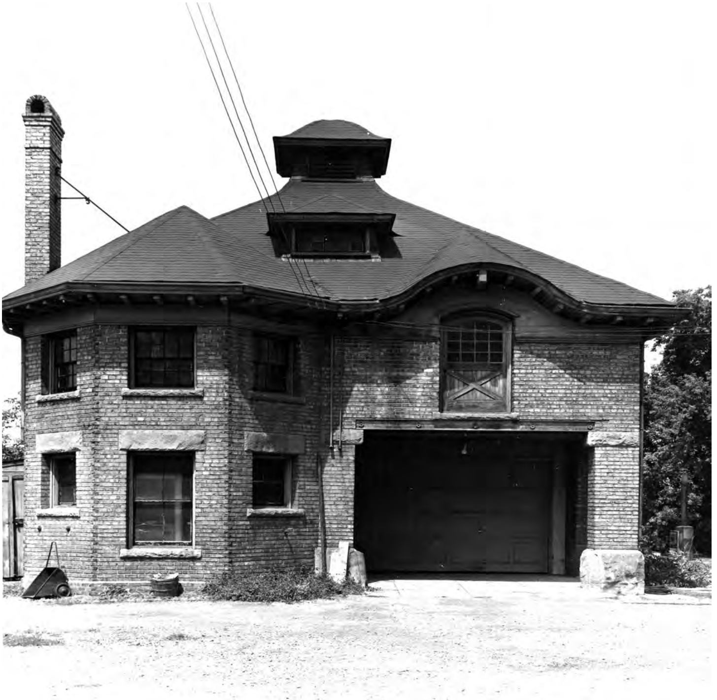
IMAGE 1: historic photo of south facade
