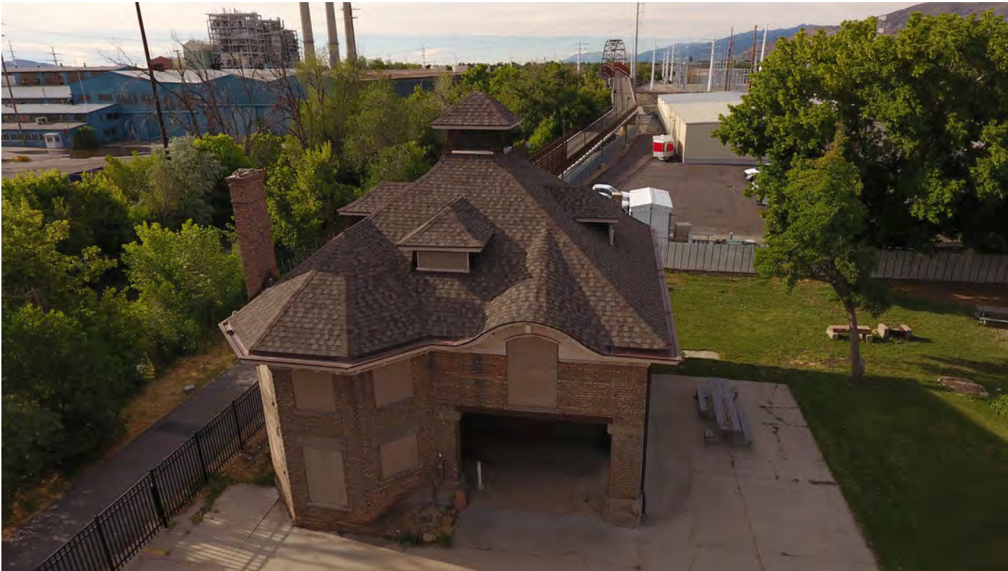
IMAGE 16: current drone aerial photo, post earthquake
