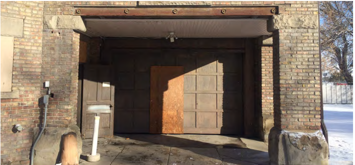
IMAGE 8: closeup of carriage entrance portico, where folding glass wall will be located, pre earthquake
