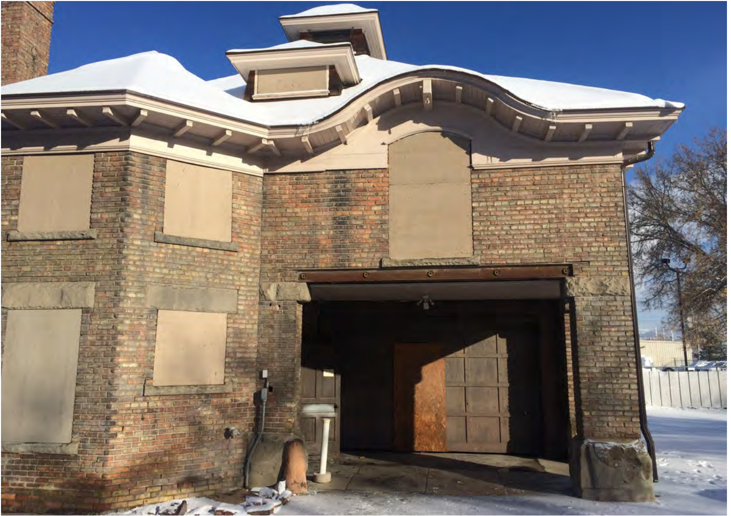
IMAGE 7: current phot of south facade, pre earthquake
