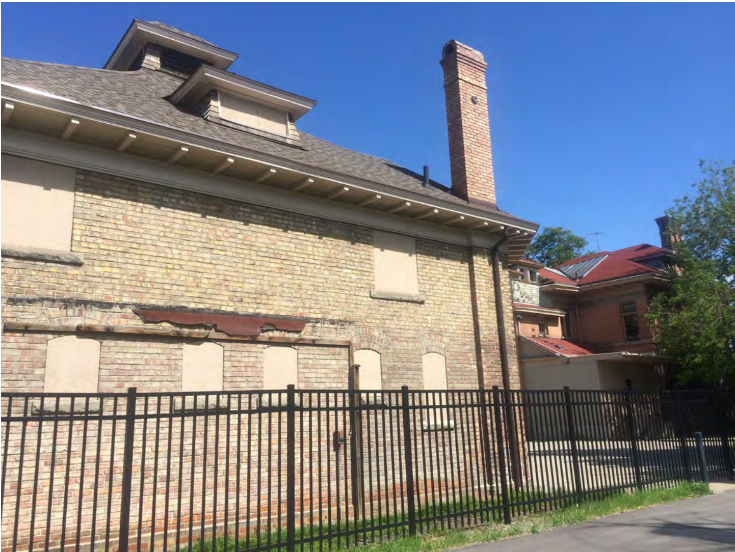
IMAGE 14: current photo of west facade, pre earthquake
