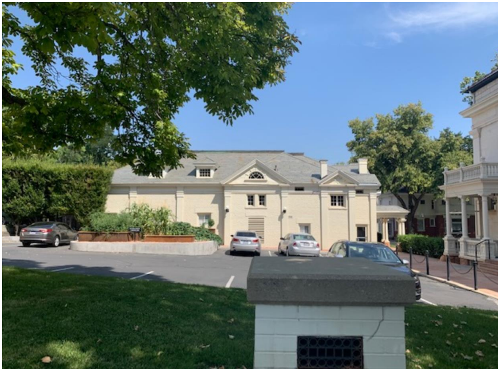
North Elevation and Carriage House
