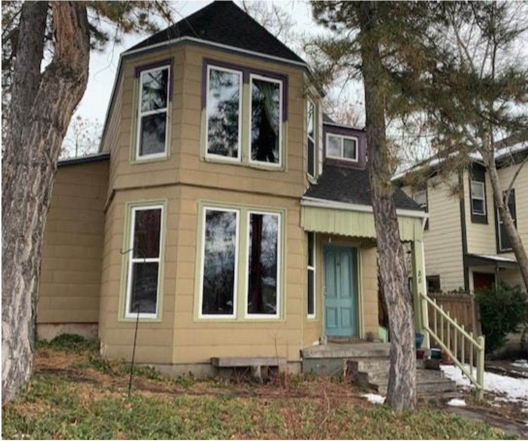
Image of the Replaced Windows
