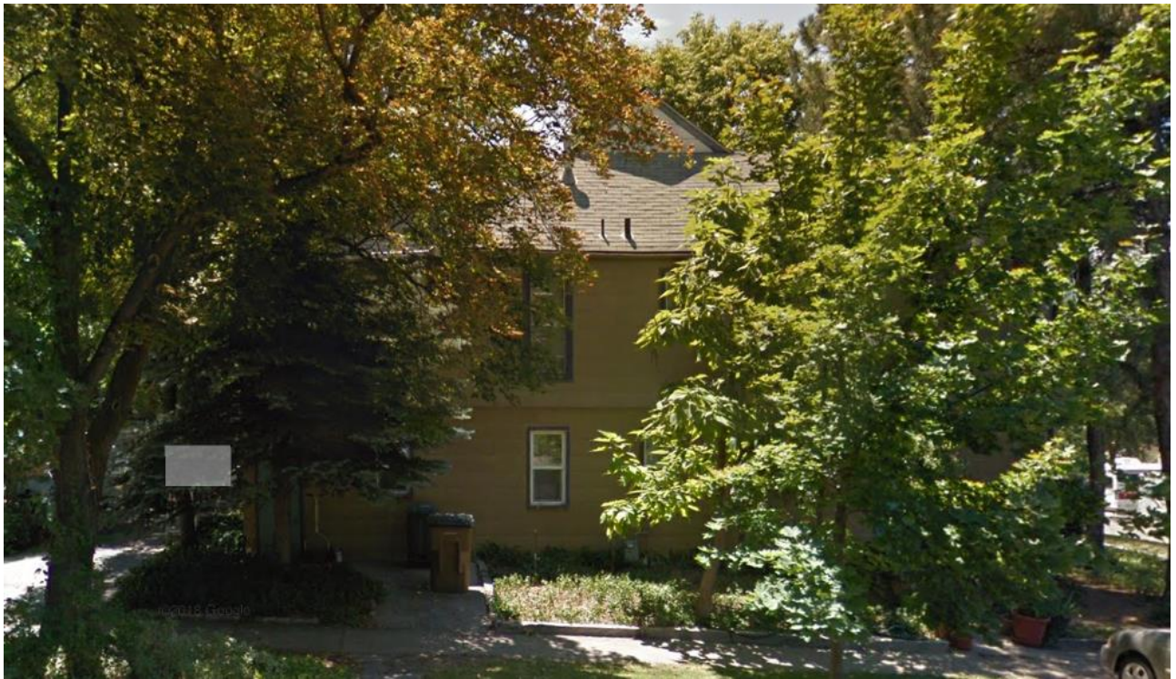
Current Image of North Elevation
