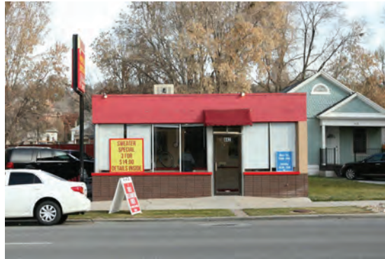
442 N. 300 W. BUILDING 2 NORTH OF PROJECT SITE
