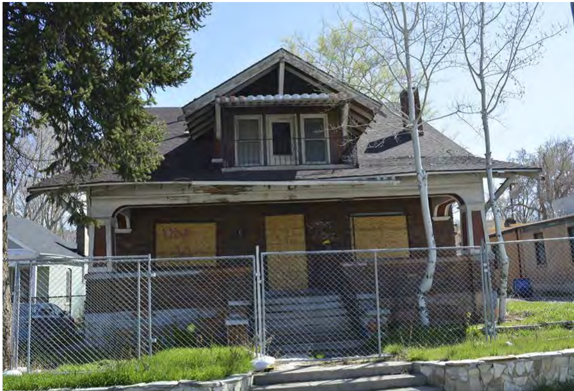
Existing home fronting on 300 West.
