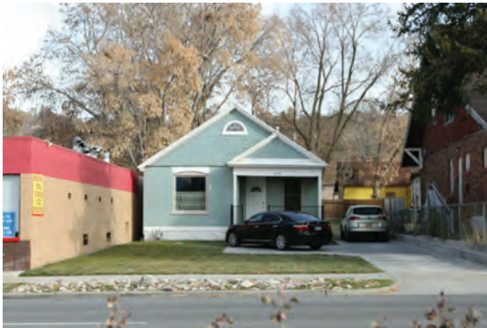
438 N. 300 W. HOME NORTH OF PROJECT SITE
