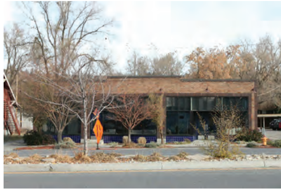
422 N. 300 W. BUILDING SOUTH OF AND IN FRONT OF PROPOSED PROJECT
