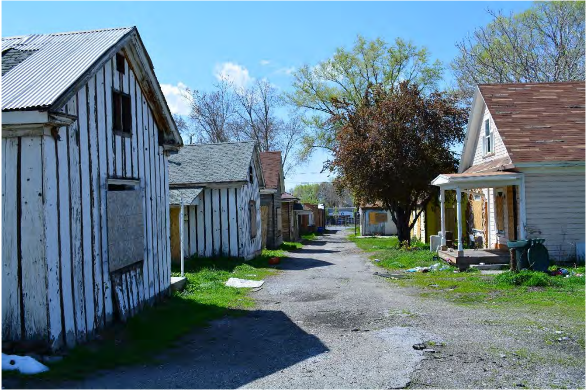
View of Bishop Place looking toward 300 West.
