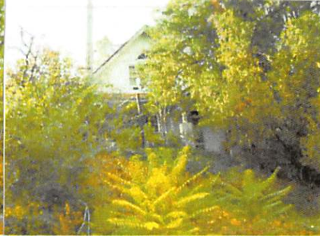
1116 East 300 South Masonry, pattern book, 1895 Hip roof with gabled projecting porch roof, fishscale shingles in gable ends, also large Palladian win- dows, brick exterior; transomed door and window.
