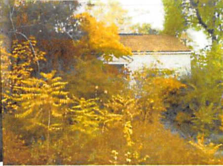
1108, 1112, and 1114 East 300 South Frame, builder's vernacular, 1895 Gable roof parallel to street, gabled porch with paired square column, stucco exterior, scalloped trim under eaves.
