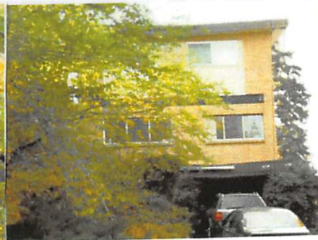
1154-56 East 300 South Masonry, apartment (1970 ?) Concrete foundation, parking under building; win- dow, aluminum slides; low pitched gable roof.
