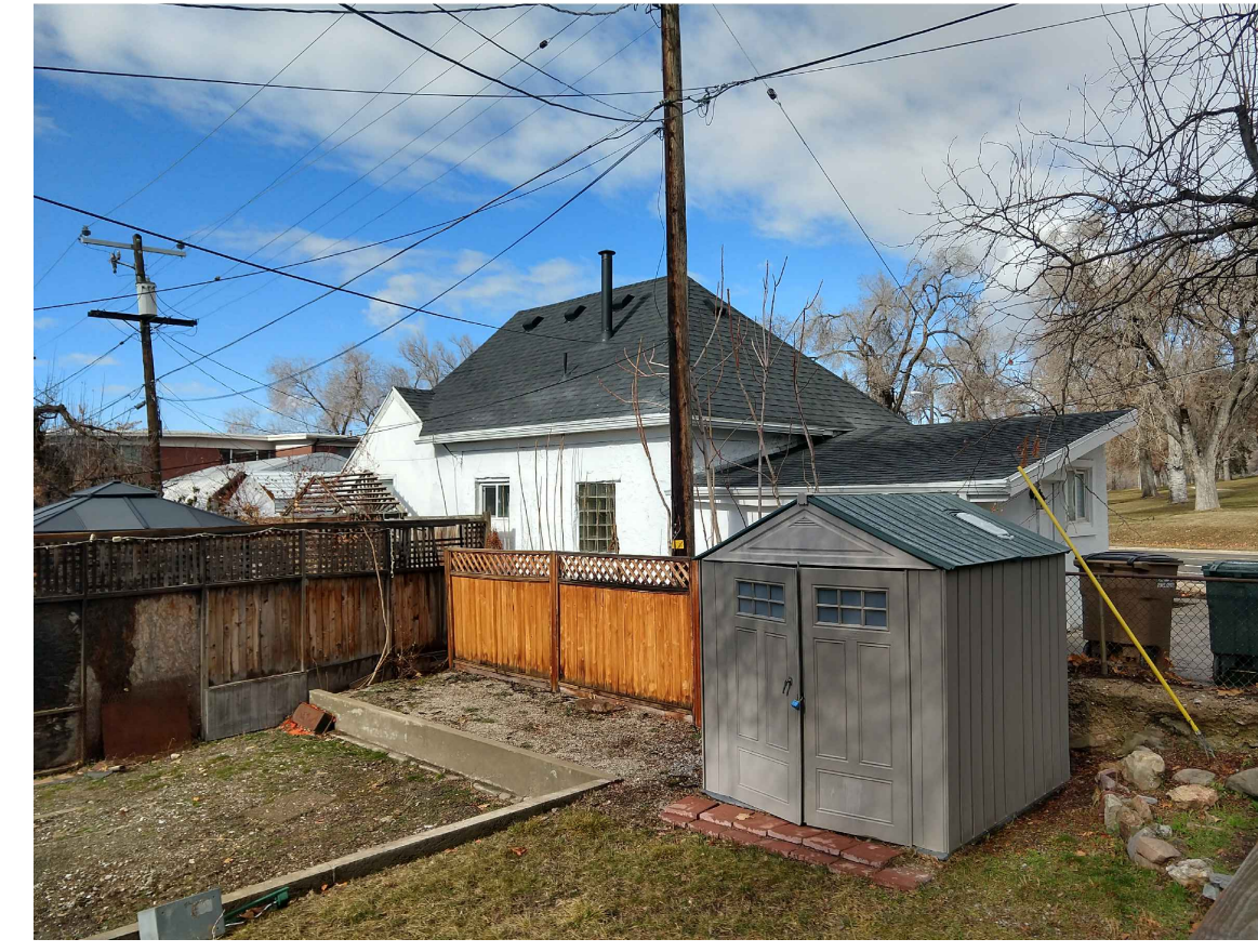
SOUTH FACING FACADE
