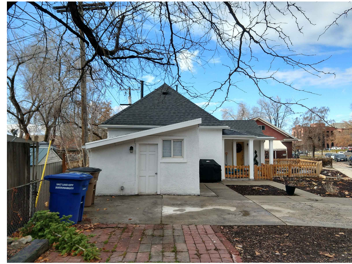
EAST FACING FACADE
