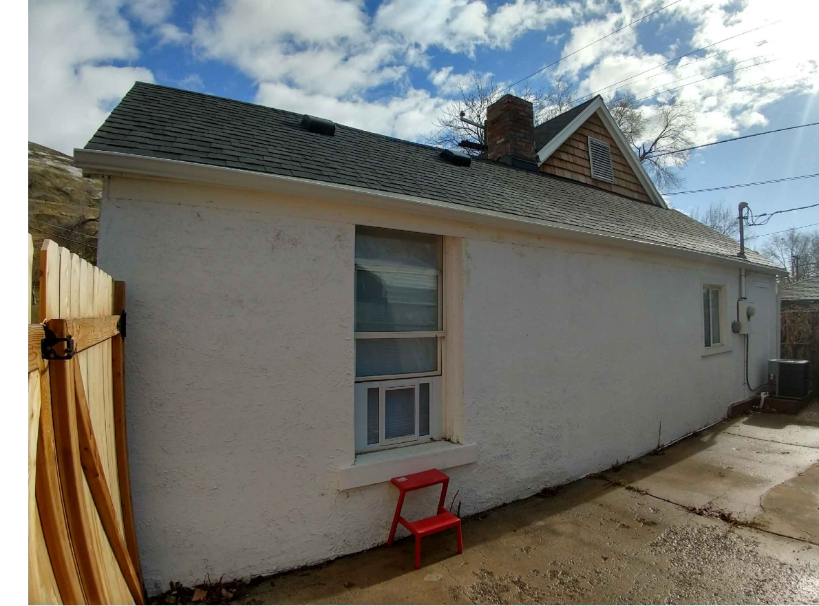
WEST FACING FACADE
