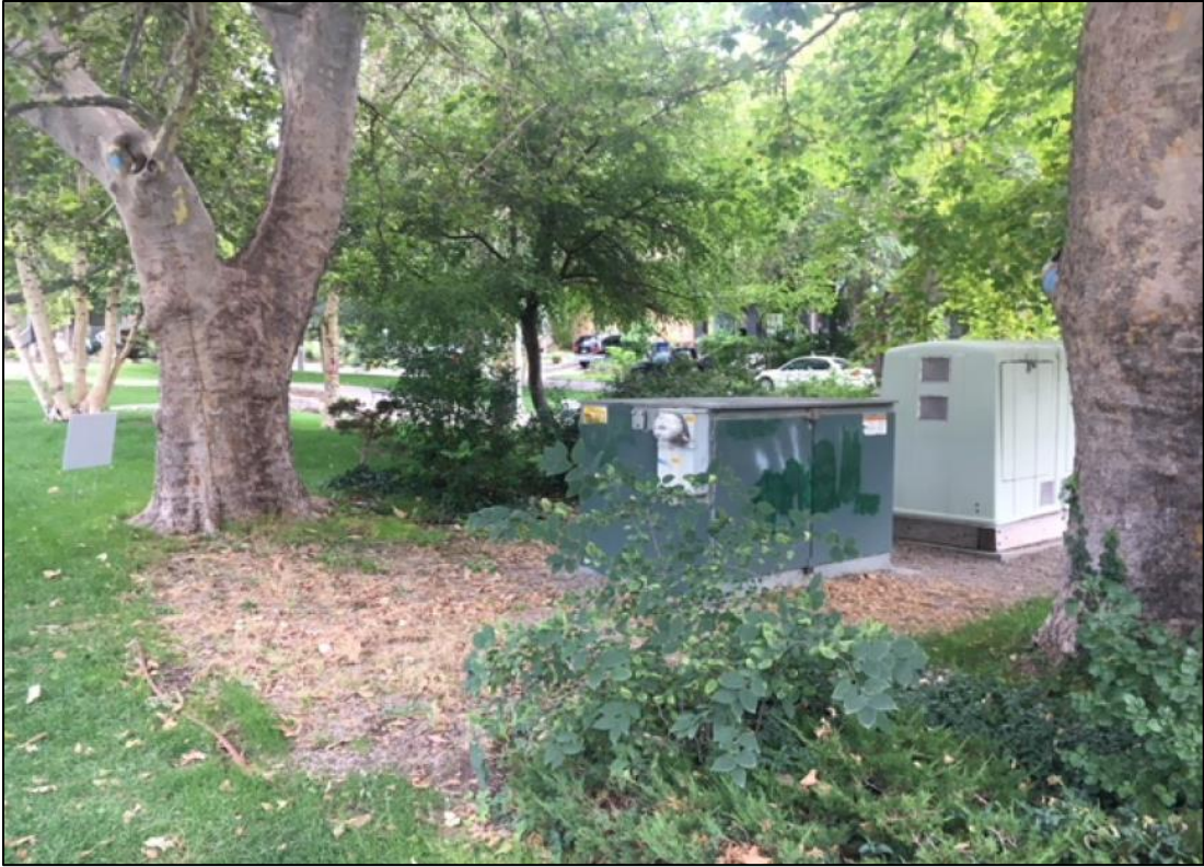
North/Eastern View of Existing Well
