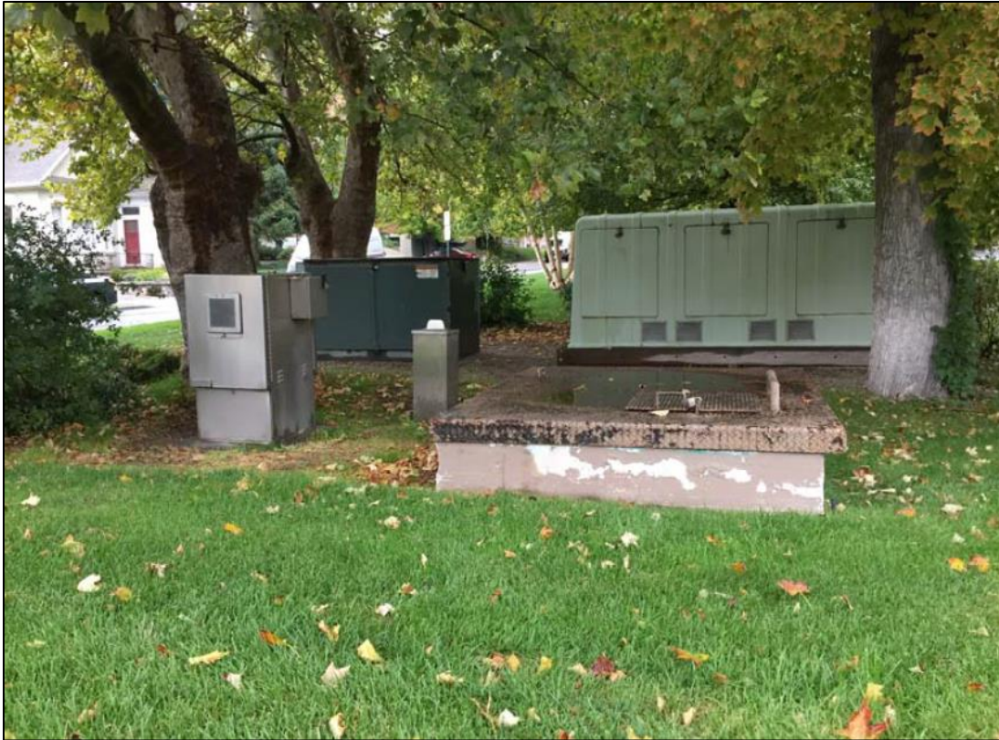
View of the Existing Well
