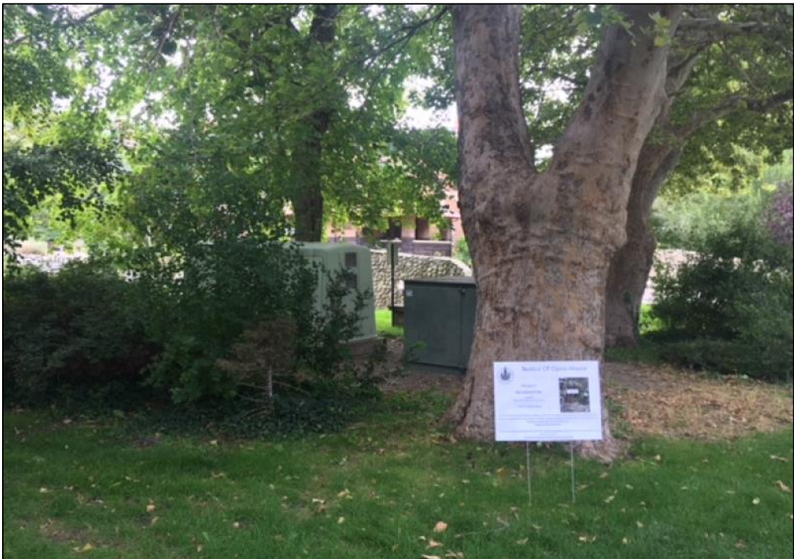
South/East View of Existing Well
