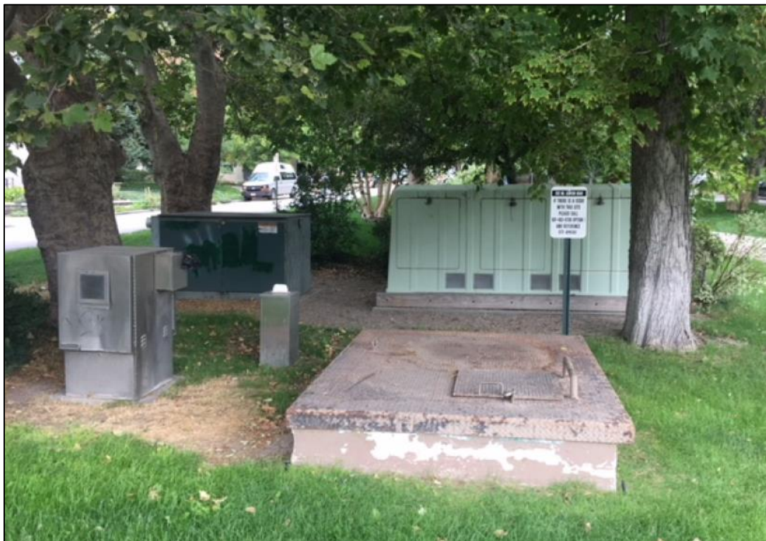
View of Existing Well
