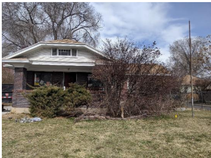
Figure 20 – Front of home at 633 E 800 S
