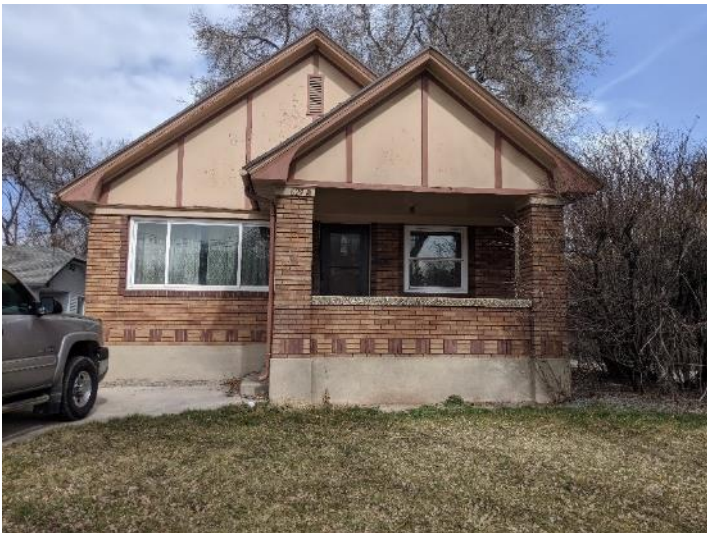
Figure 17 – Front of home at 629 E 800 S
