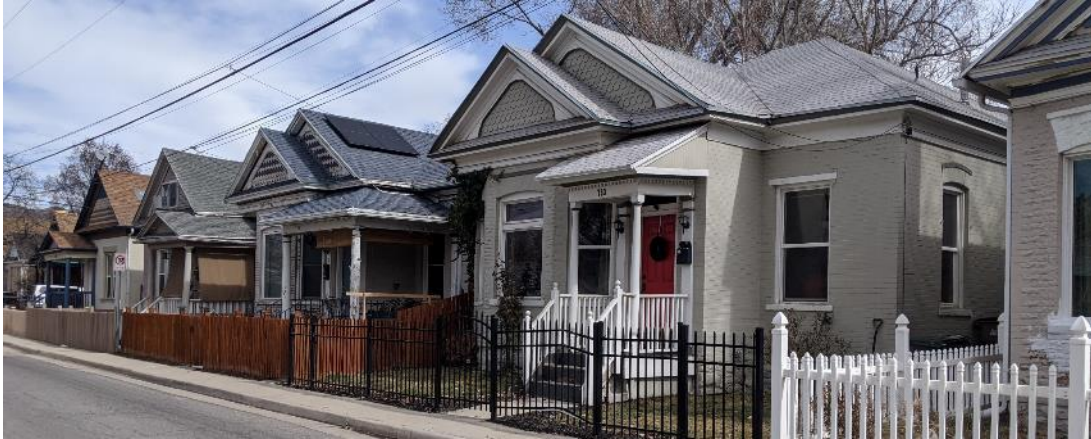
Figure 7 – Homes located on the east side of Green Street.
