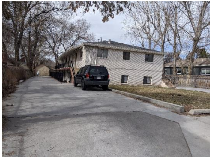
Figure 23 – Existing apartment building to the north of 633 E 800 S
