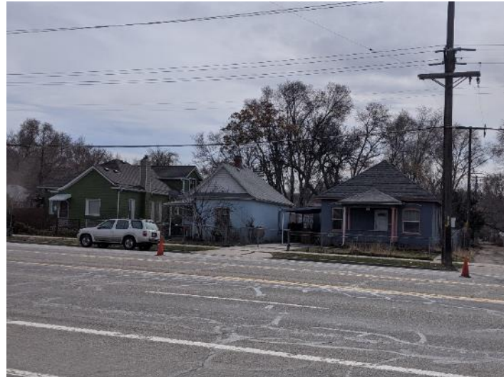
Figure 25 – Homes on the south side of 800 S
