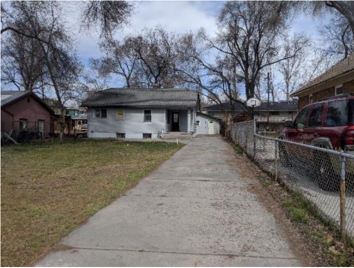
Figure 16 – Front of home at 625 E 800 S
