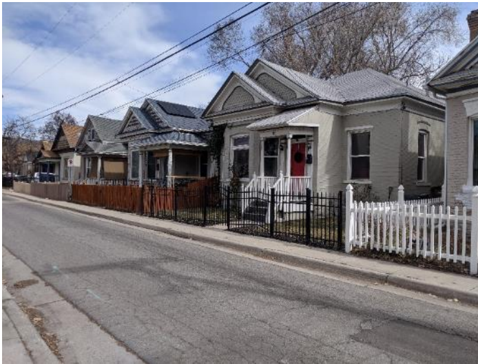
Figure 24 – Homes on the east side of Green Street
