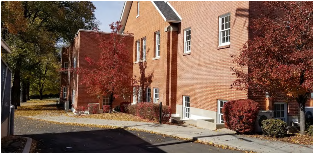
Existing south side, east end
