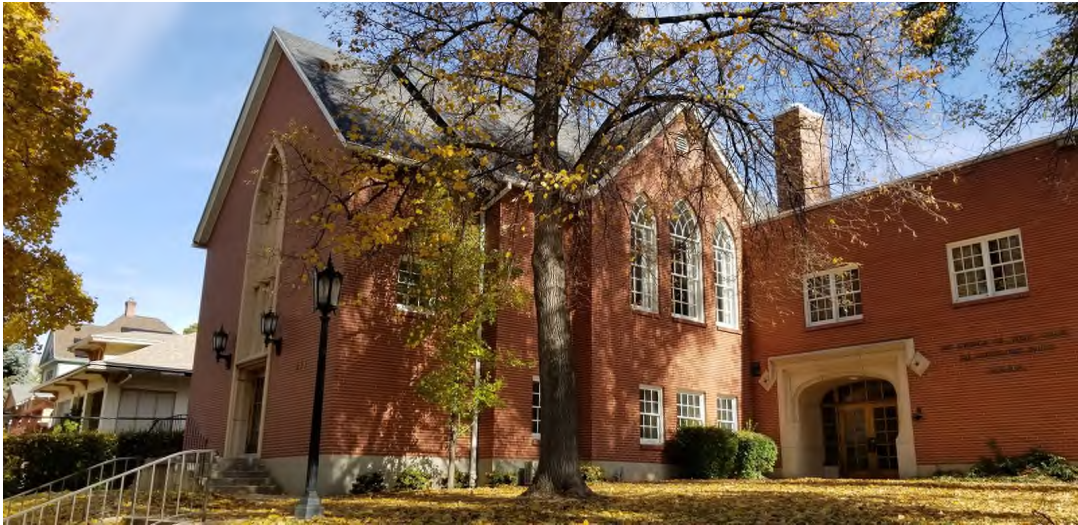
1100 East (west) view of building at sidewalk level
