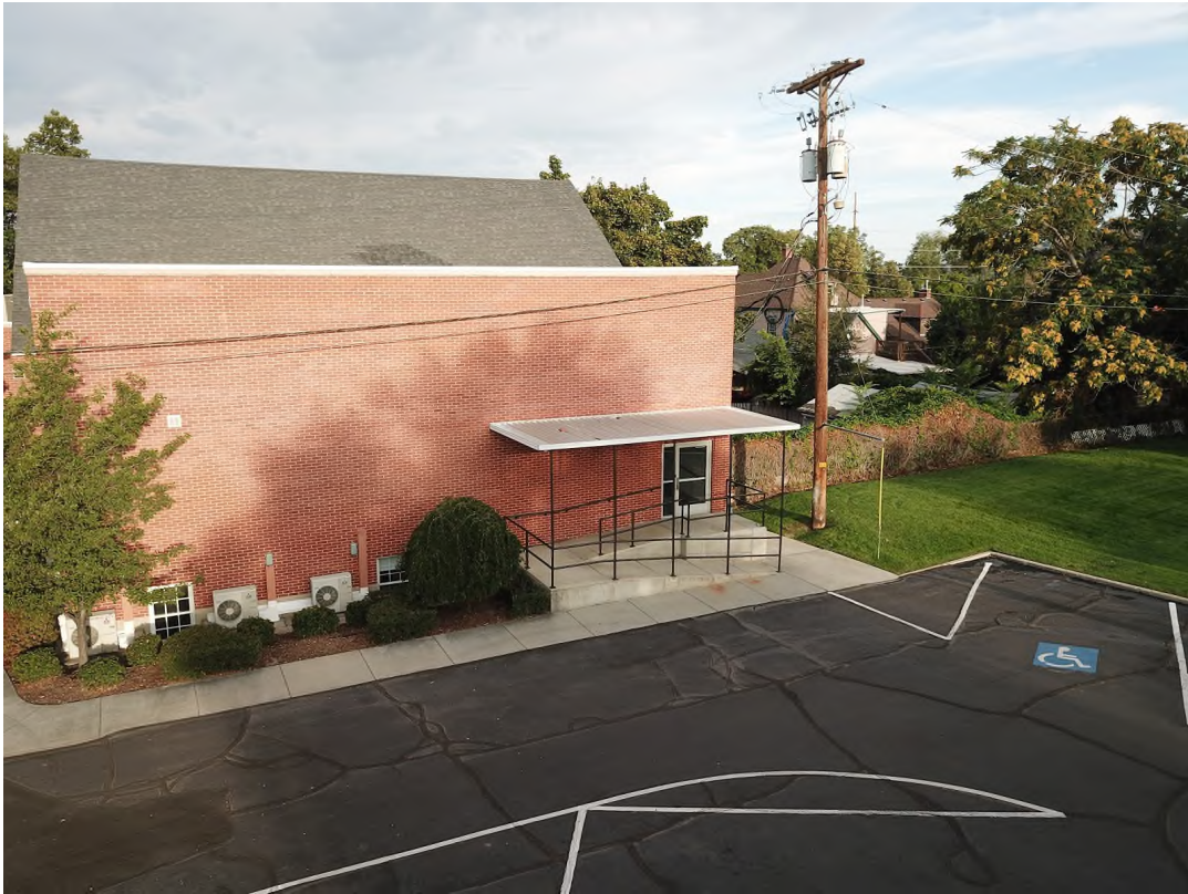
Aerial view of Existing Building, east entry and ramp area
