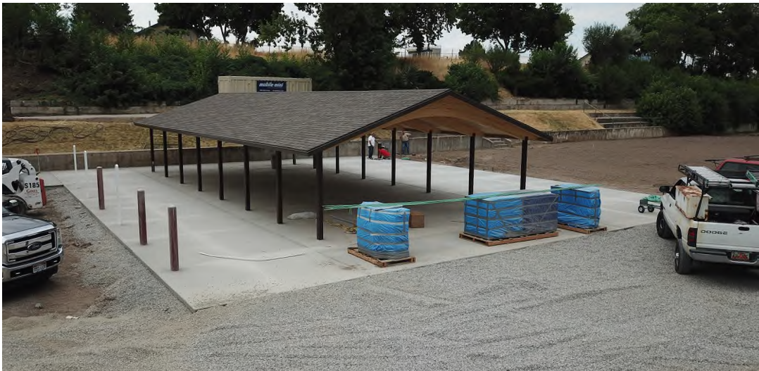
Photograph of similar pavilion structure: Shingle roof, exposed wood beams and steel posts
