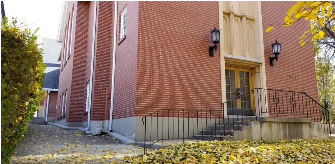
Existing west side, north end
