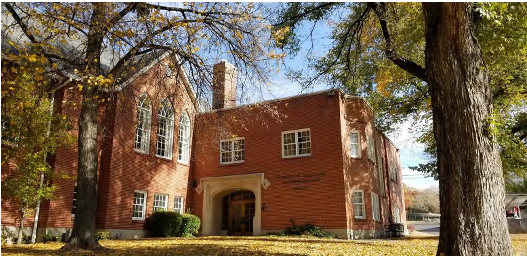
Existing west side, south end
