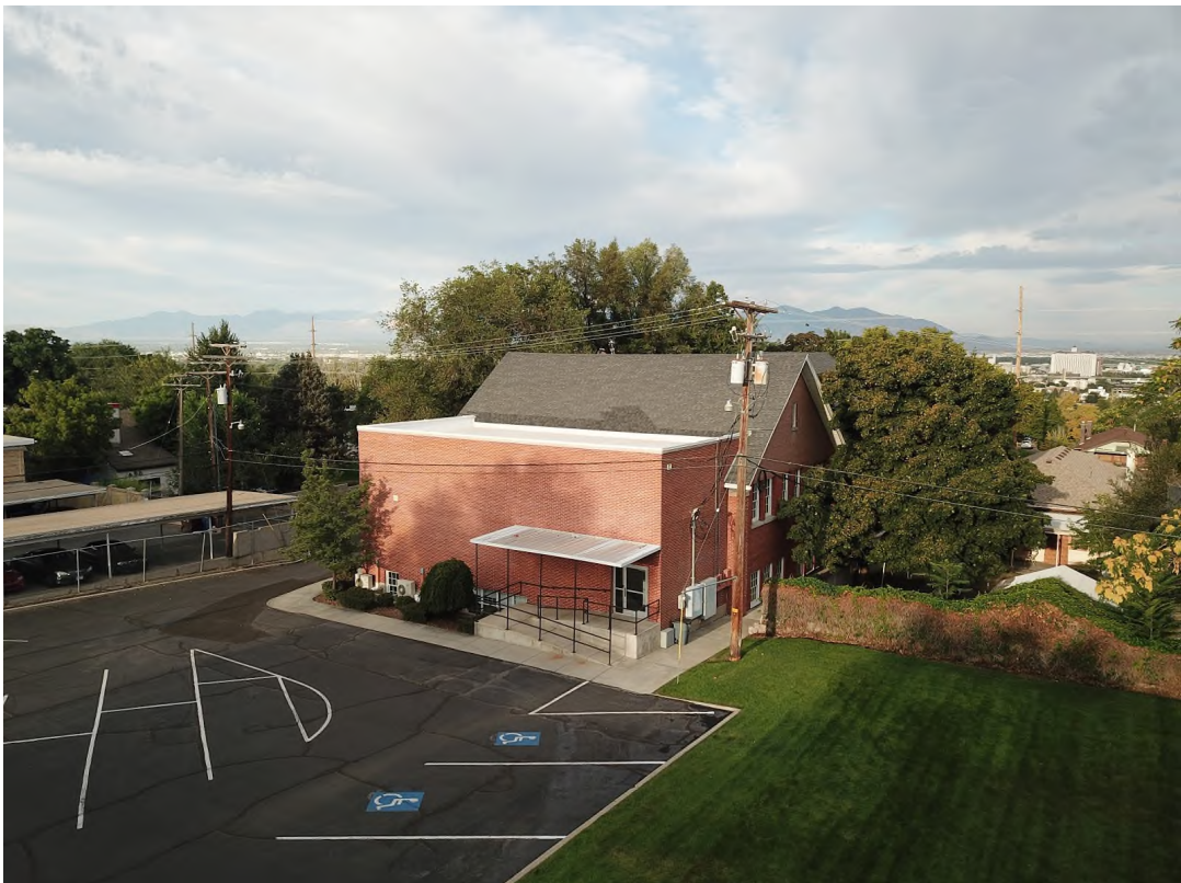
Aerial view of existing building from northeast
