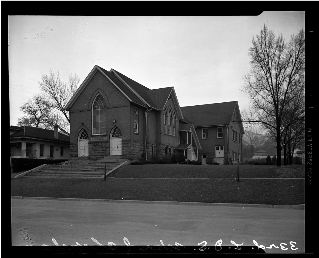
West side (1100 East) of original building Source: Utah State Historical Society
