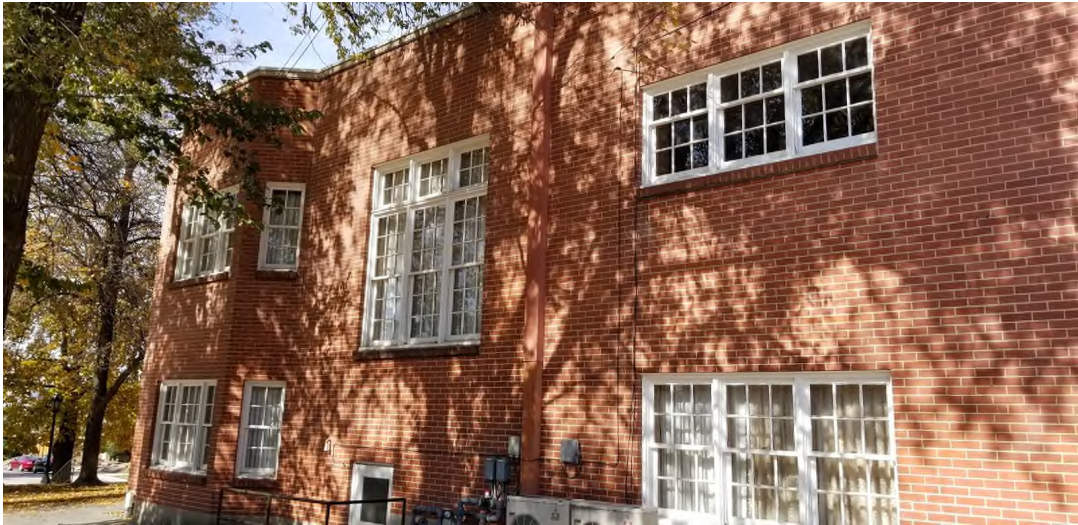
Existing south side, west end
