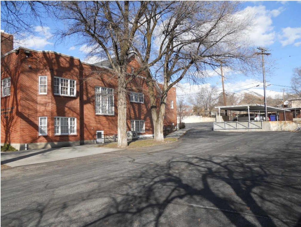
The view toward the rear of the building as seen from the existing parking lot.
