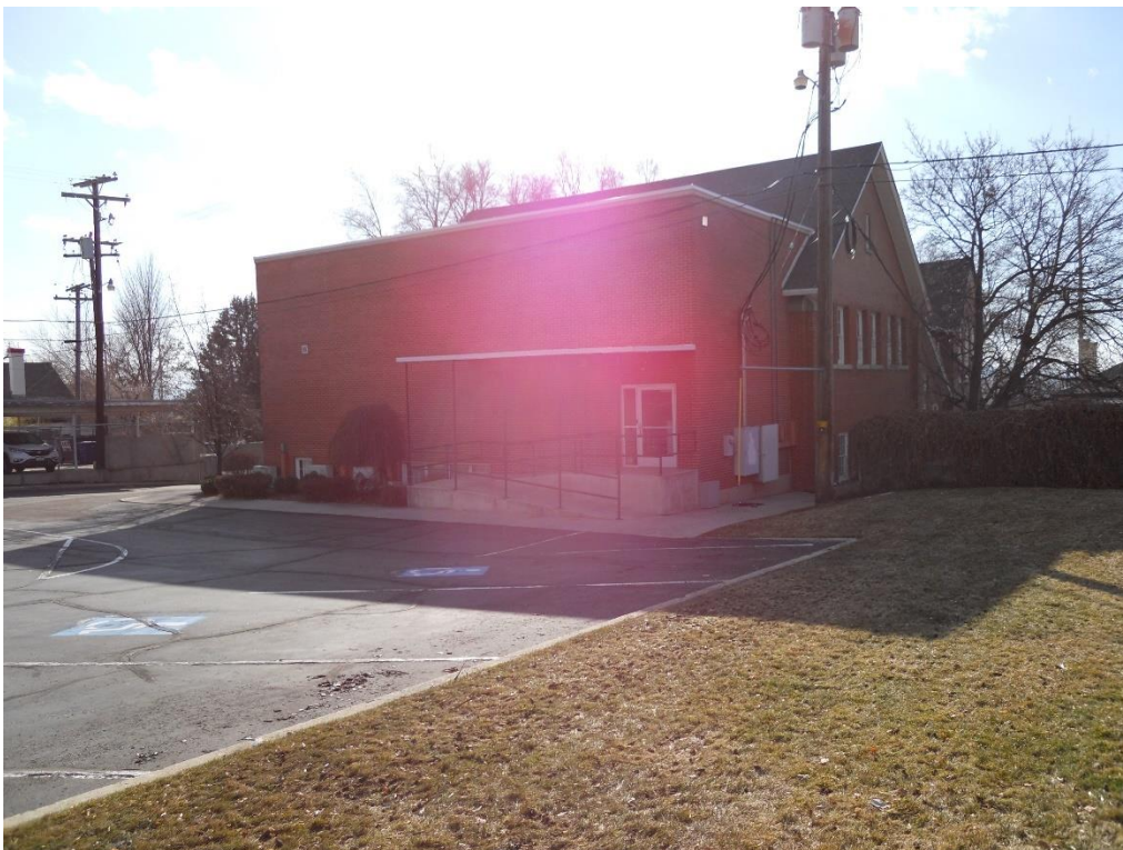
The rear of the meeting house and the ADA access to be rebuilt and improved.
