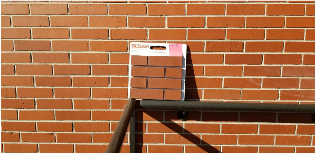
New brick veneer to match existing appearance
