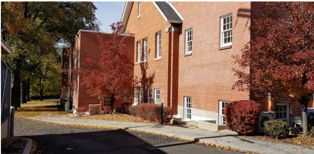
Existing south side, east end
