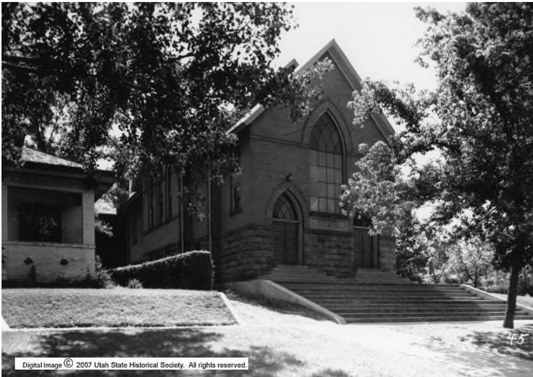
West side (1100 East) of original building Source: Utah State Historical Society
