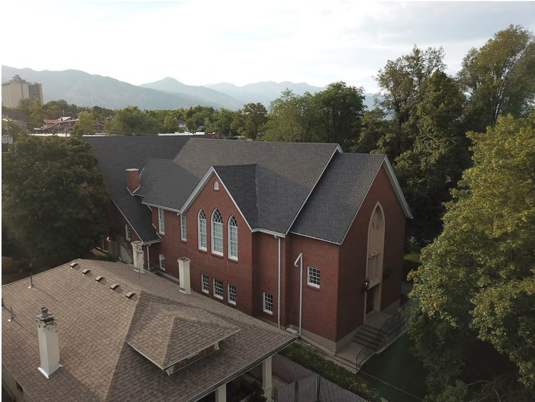
Aerial view of Existing Building, north and west sides
