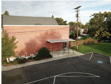
EXISTING CANOPY AND RAMP AREA
