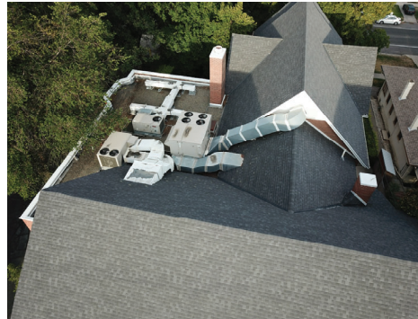
EXISTING ROOF AT NEW ELEVATOR AREA
