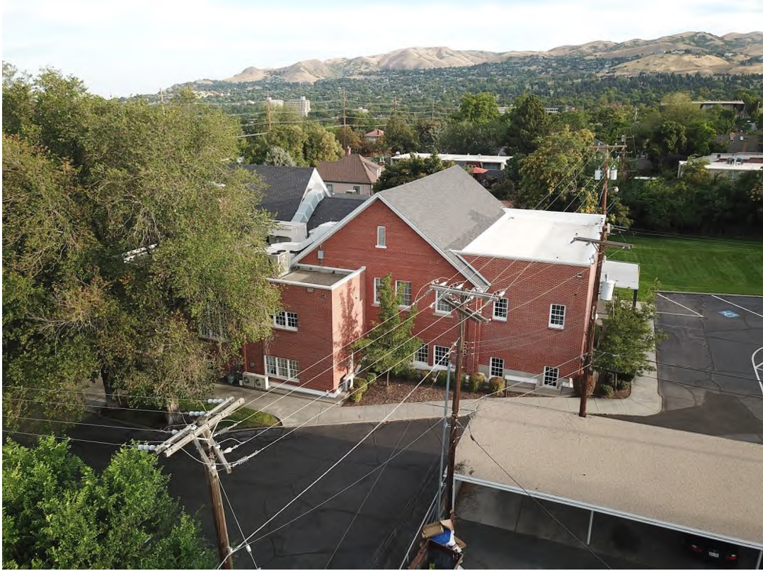
Aerial view of Existing Building, from south
