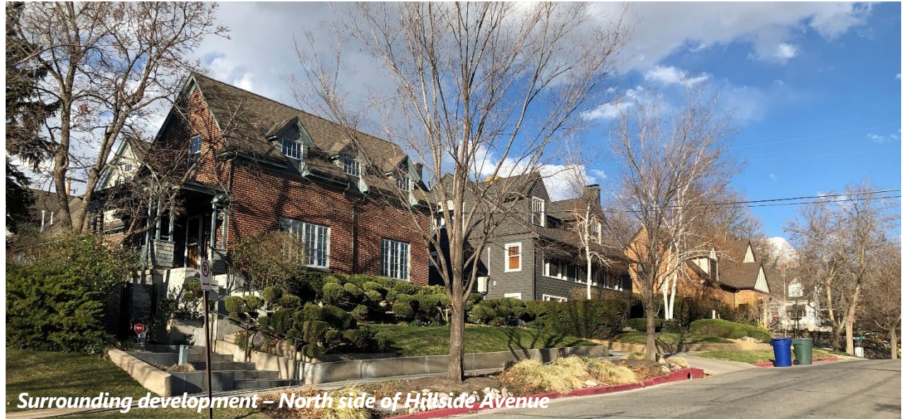
Surrounding development – North side of Hillside Avenue
