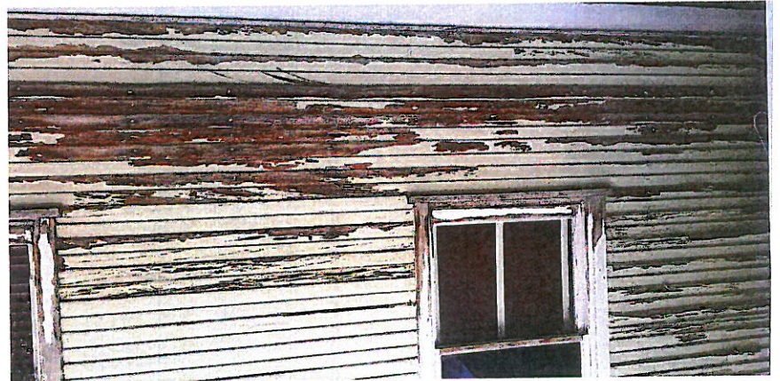
4/A NOT SALVAGABLE SIDING
