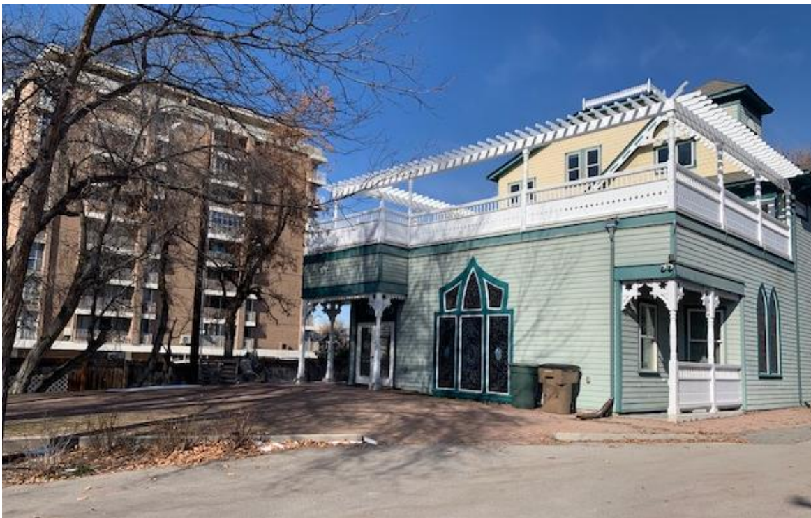
Rear of the Freeze Mansion
