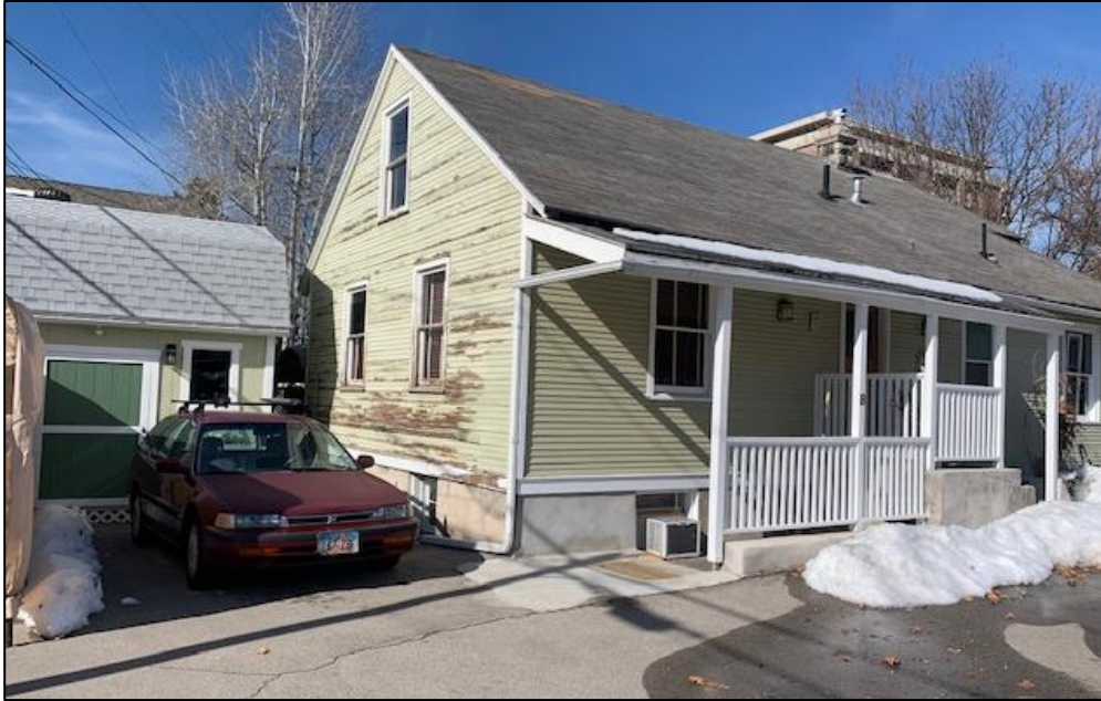
Photo of East and South Elevations
