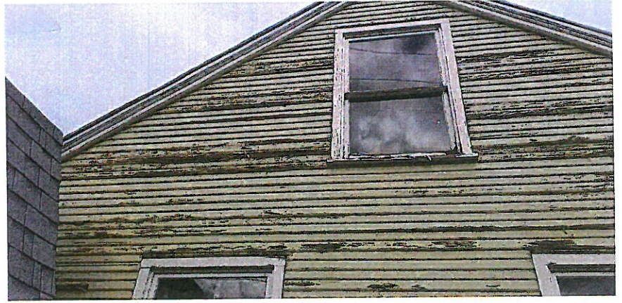
2/A SOUTH WALL-UPPER
