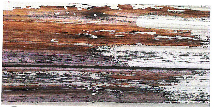
8/A DETERIORATED LAPBOARD
