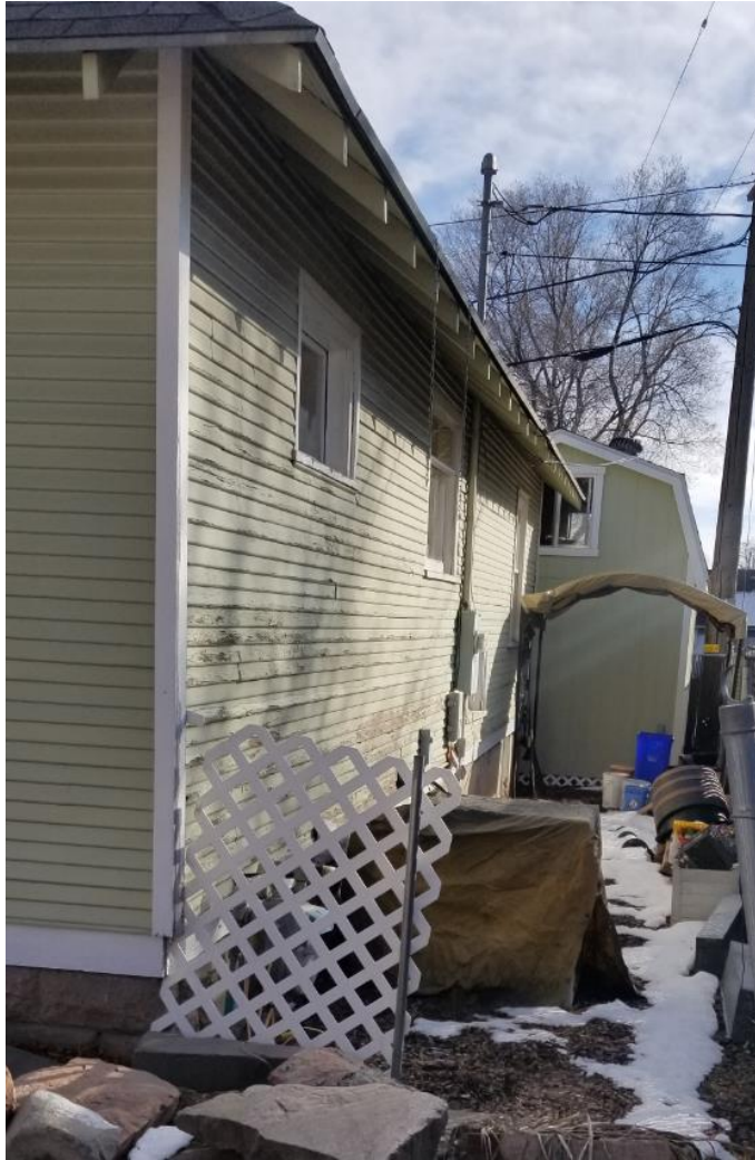
Photo of West Elevation
