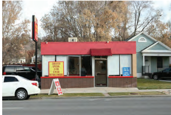
442 N. 300 W. BUILDING 2 NORTH OF PROJECT SITE
