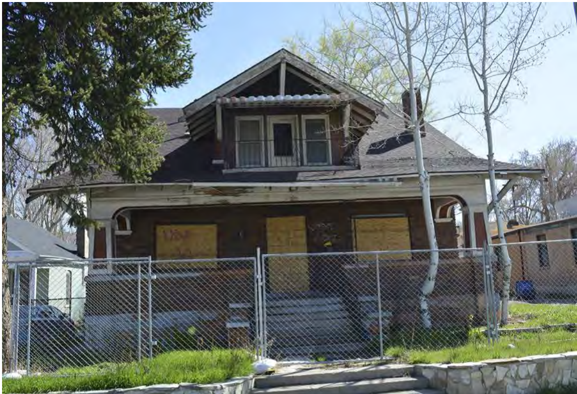
Existing home fronting on 300 West.
