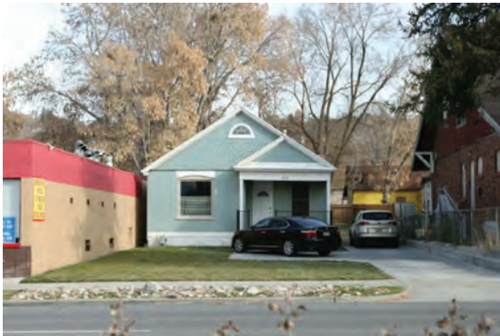
438 N. 300 W. HOME NORTH OF PROJECT SITE
