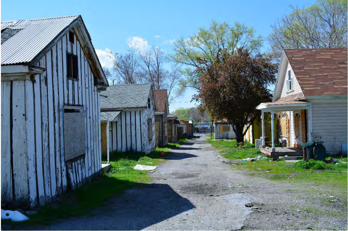
View of Bishop Place looking toward 300 West.
