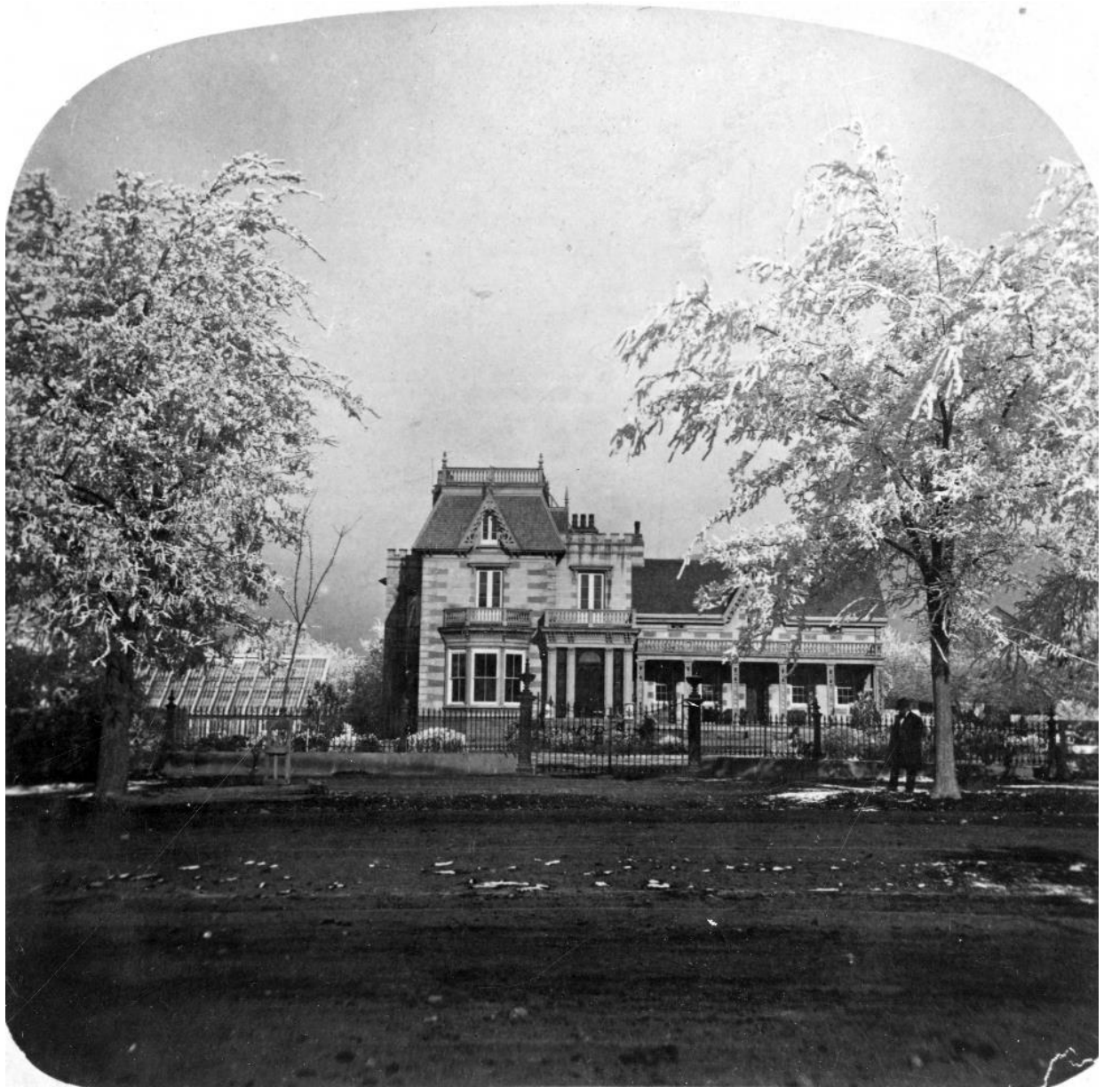
House with first addition – c. 1874, the Staines Cottage is the 1 ½ story side gabled area on the right. Source: USHS
