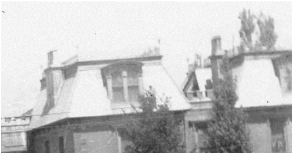
Inset of above photo shows dimensioning, shape, and coloring similar to slate
