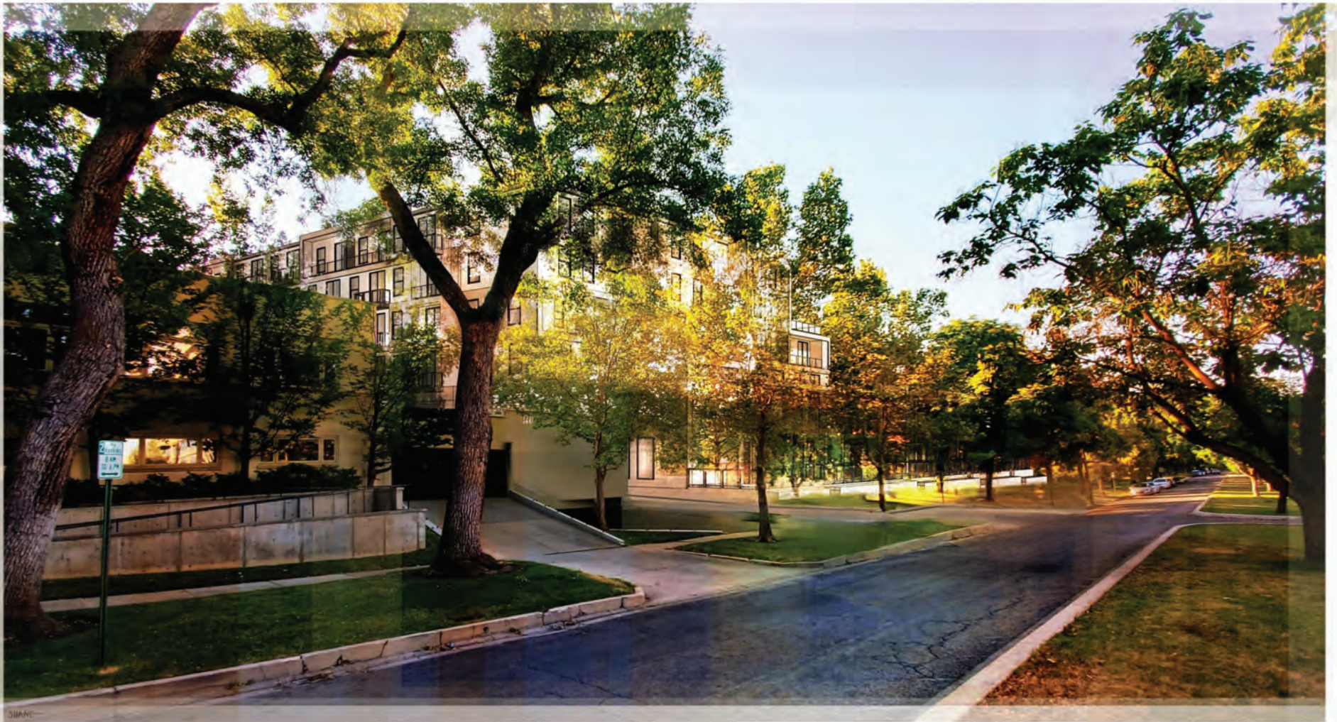
NORTHWEST STREET VIEW
