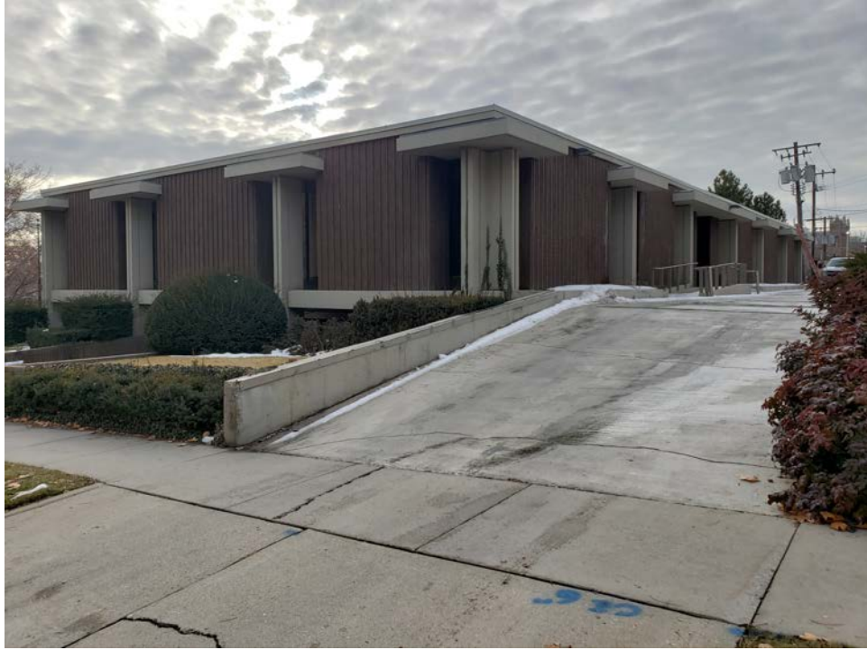
Photograph 12 of 29 North and east elevation of Steiner American Building. Camera facing southwest
