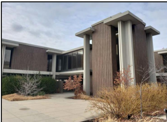
South and east elevation of Steiner American Building. Camera facing northwest – 2019.
