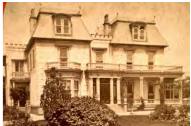
Figure III-10. A view of the Devereux House about 1880.
