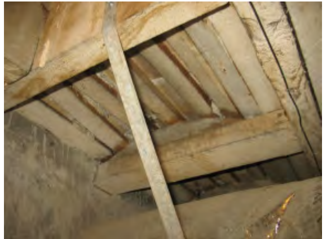
Figure III-29. Floor framing underneath the fireplace hearth in the Library.
