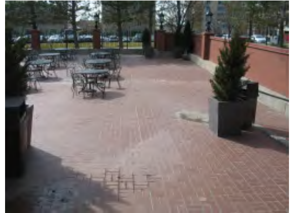
Figure IV-38. A view of the patio surface.
