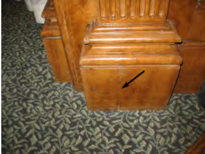
Figure III-36. A pilaster base showing a splice where a repair was inserted.
