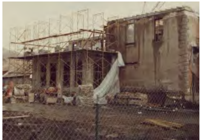
Figure III-23. A view of the west elevation during construction in 1983.
