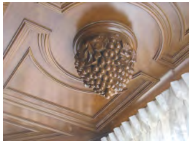
Figure III-39. The grapevine cluster and wood soffit after restoration.
