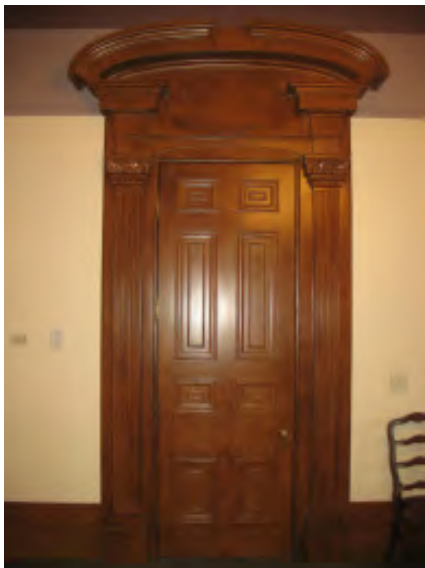
Figure III-41 (left). The door leading to the Stair Hall.
