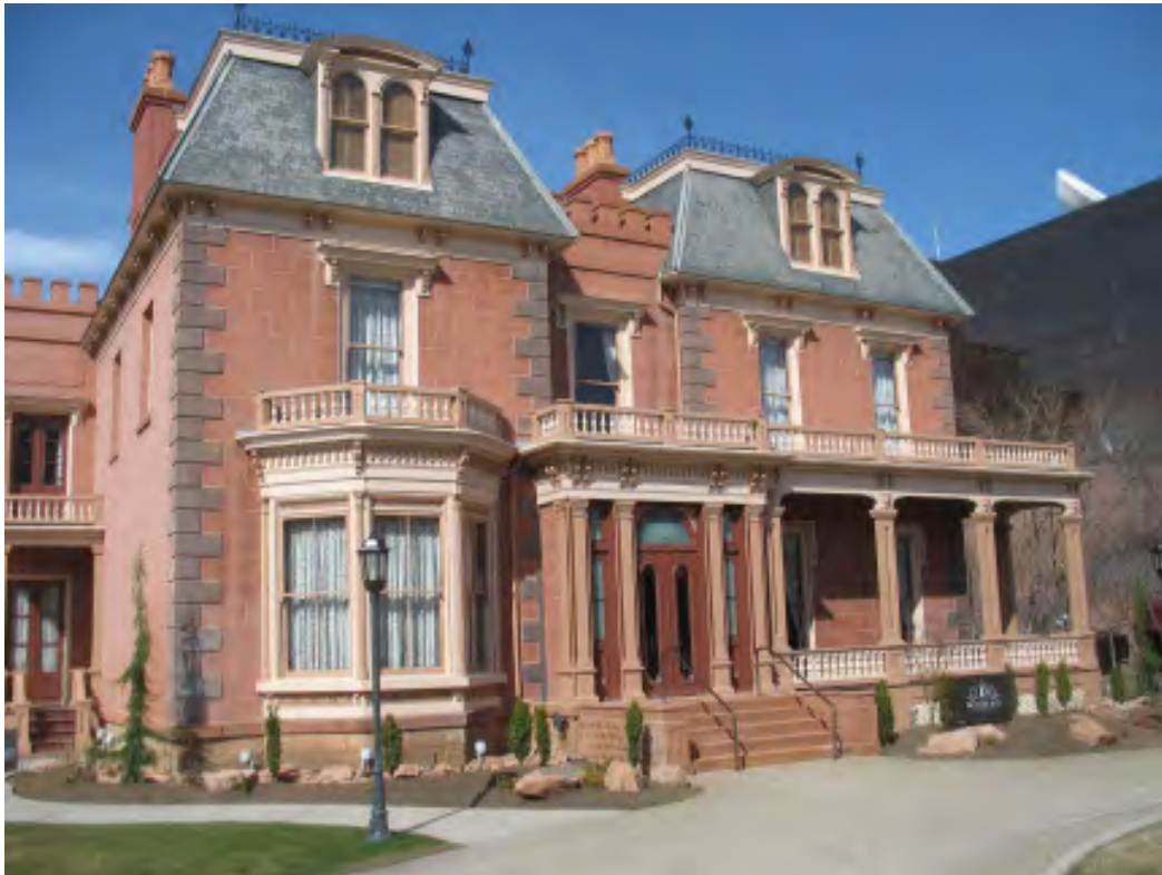
Figure III-1. The south elevation of the Devereux House.
