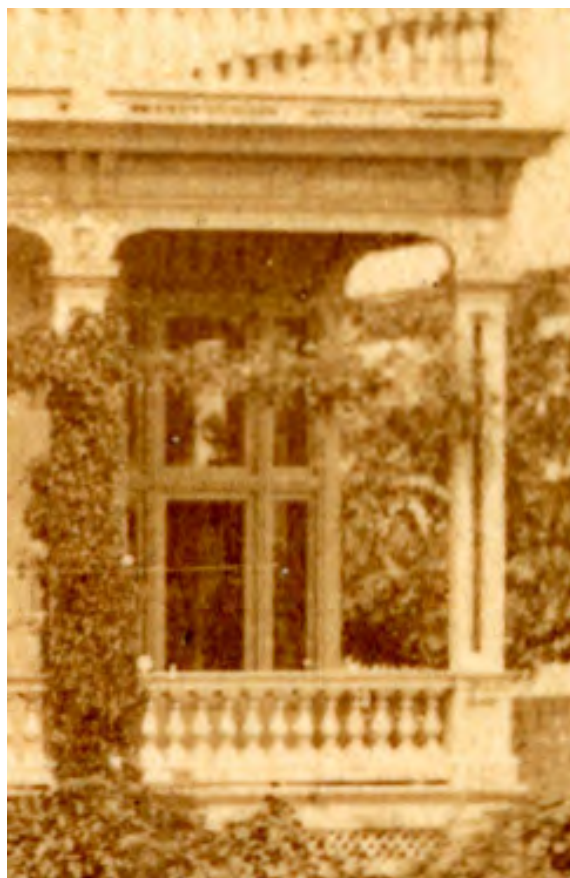
Figure II-9 (left). A detail from an 1880 photograph showing the Conservatory tucked underneath the porch roof.
