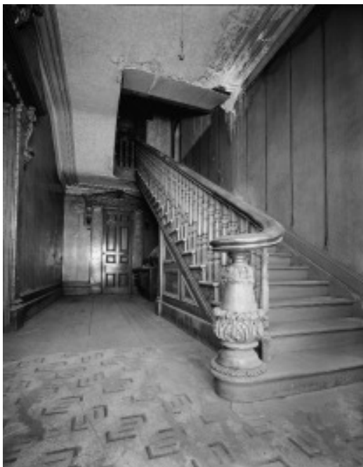
Figure III-45 (left). The Stair Hall in 1967, HABS #U-37, photo #2.
