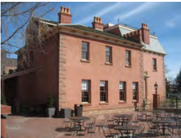
Figure III-22. The west elevation of the Devereux House.
