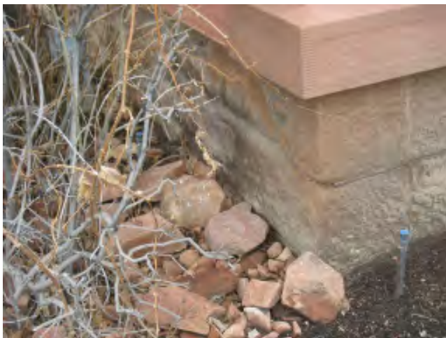
Figure IV-1. A detail of the southwest corner of the Devereux House foundation.
