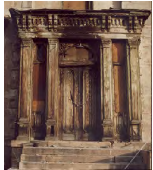
Figure III-3. The entrance pavilion before restoration.
