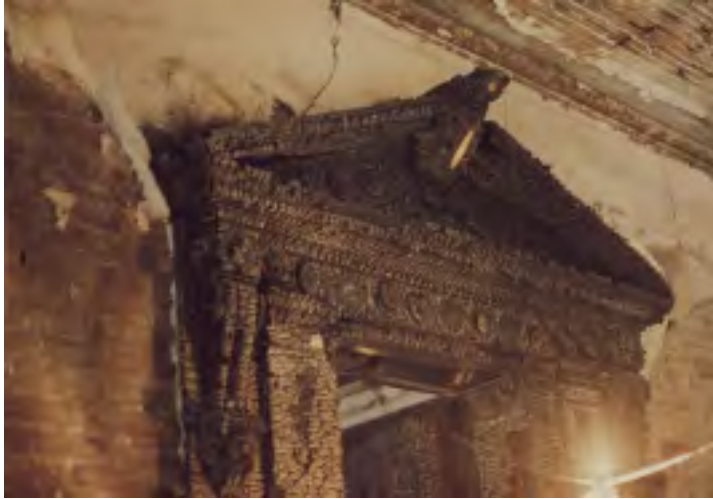
Figure III-47 (above). A photograph of a charred doorway in the Stair Hall.
