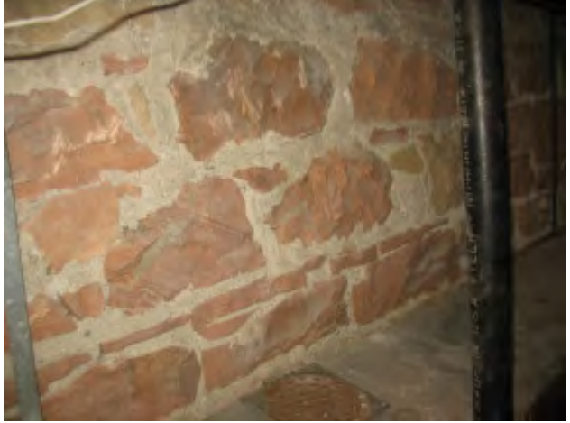
Figure III-26. A view of a typical sandstone foundation wall.
