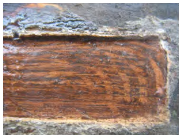
Figure III-58. A detail of the graining on the original window panel.
