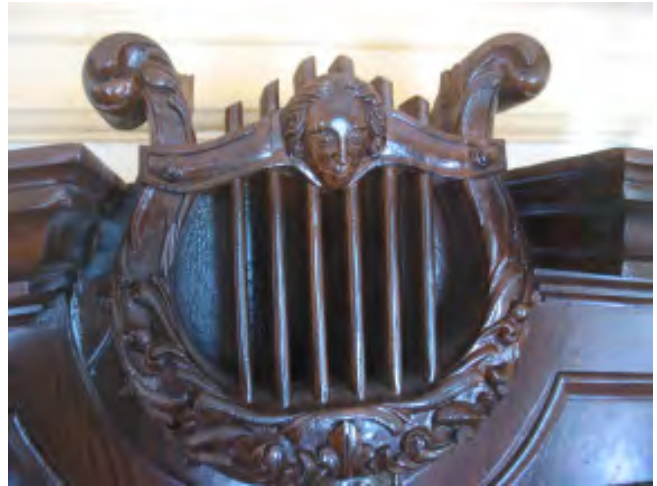
Figure III-52. A detail of the lyre in the double pocket door pediment.
