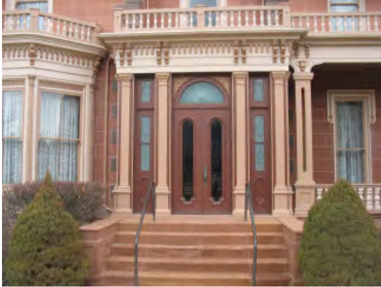
Figure III-2. The entrance pavilion on the south elevation.
