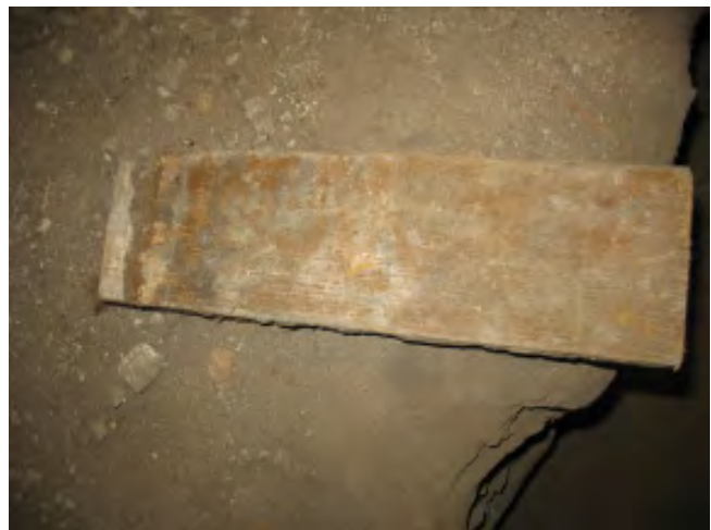
Figure III-32. A fragment of original flooring found in the crawl space.
