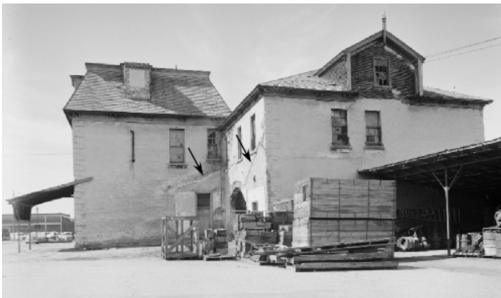
Figure III-18(left). The north elevation of the Devereux House in 1967, HABS #U-37, photo # 7. Note the outline of the missing roofs of the shed roof kitchen addition (left arrow) and the gable roofed laundry addition (right arrow).
