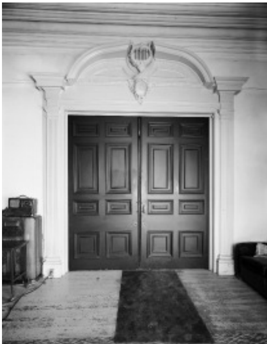
Figure III-50 (bottom) The double wide pocket doors in 1967, HABS #U-37, photo # 21.
