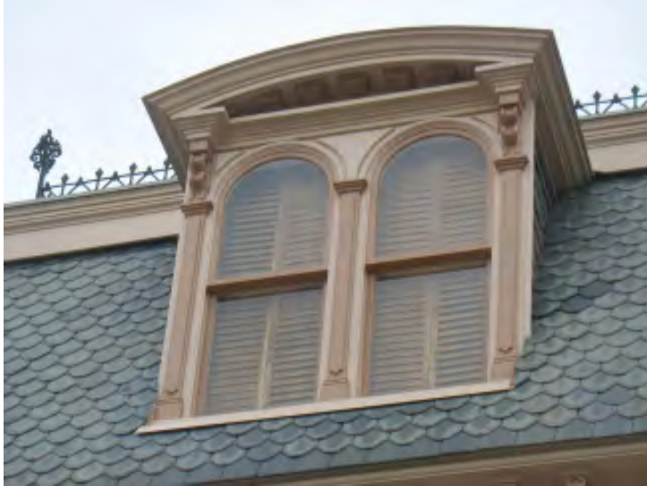
Figure III-5 (left). A mansard roof dormer.
