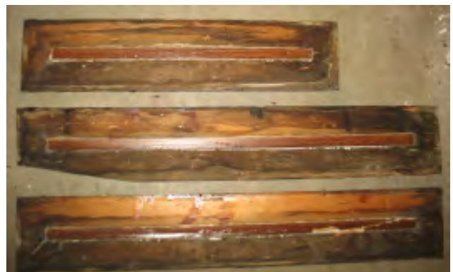
Figure V-4. The interior side of saved window panel boards
