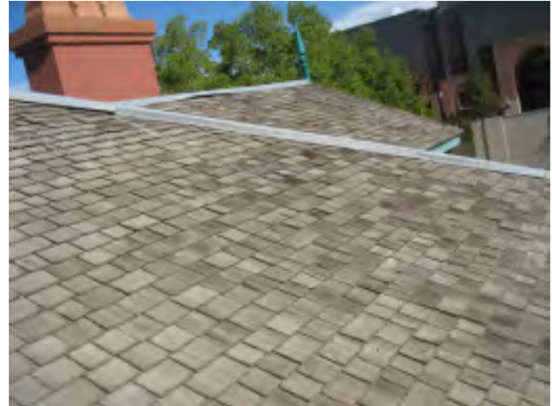
Figure IV-30. A view of the rear wing roof.
