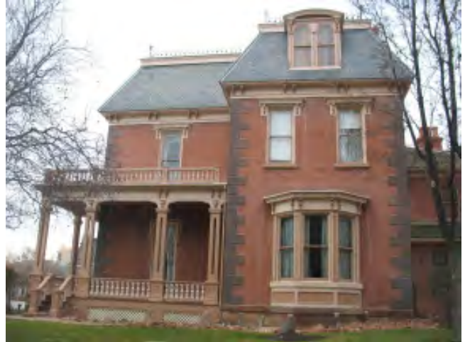
Figure III-14. A partial view of the east elevation.
