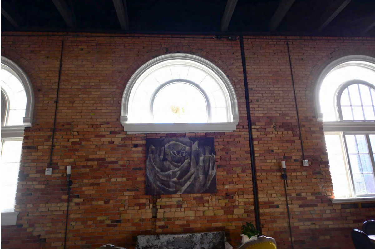
Photo No. 25 of 30, Second floor level interior. Camera facing east.
