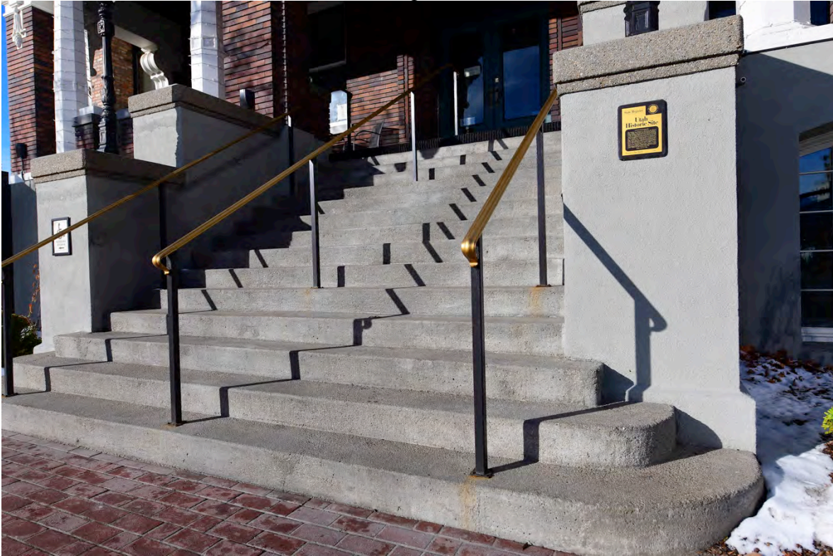
Photo No. 2 of 30, East elevation. Camera facing southwest.
