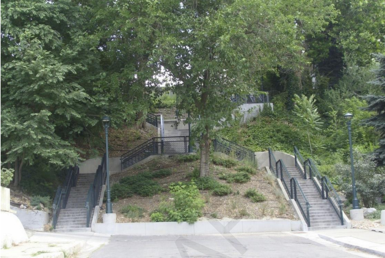
Historic Topography at 4th Avenue Stairs (photo: Landmark Design)
