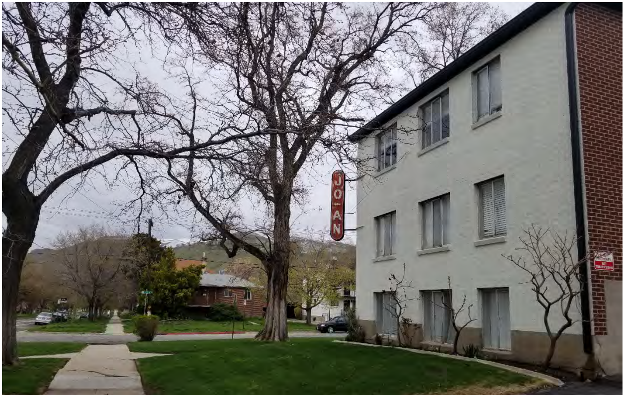
Image 11 – West façade of the building after paint was applied
