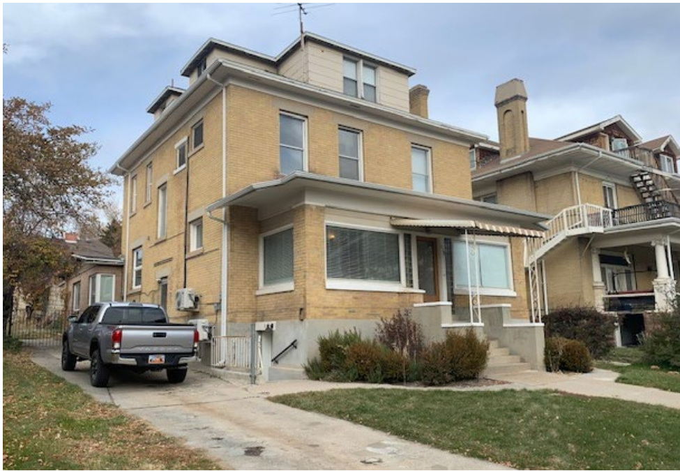
West and Southern Elevation of 679 2nd
