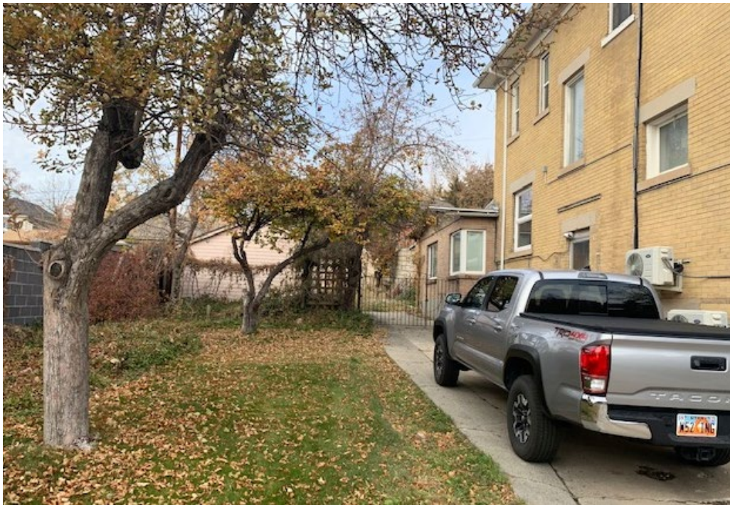
West Elevation of 679 2nd
