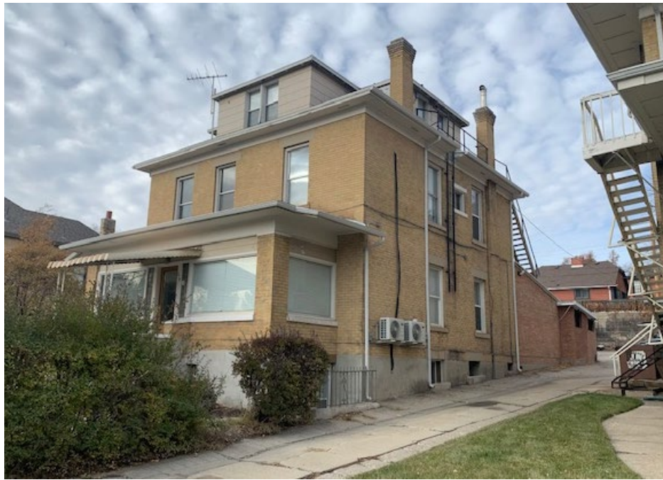
Eastern Elevation of 679 2nd
