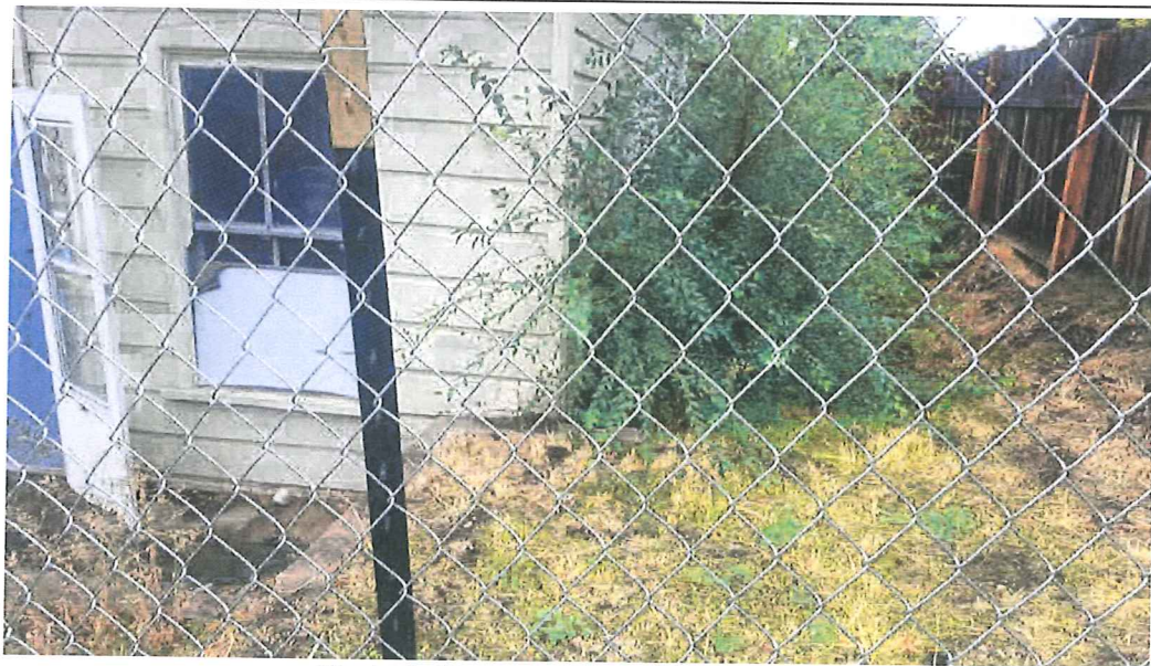
Photo 4: Home constructed below grade.
