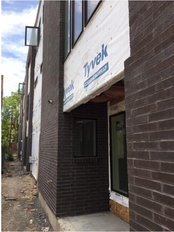
Back Stoop On West Façade
