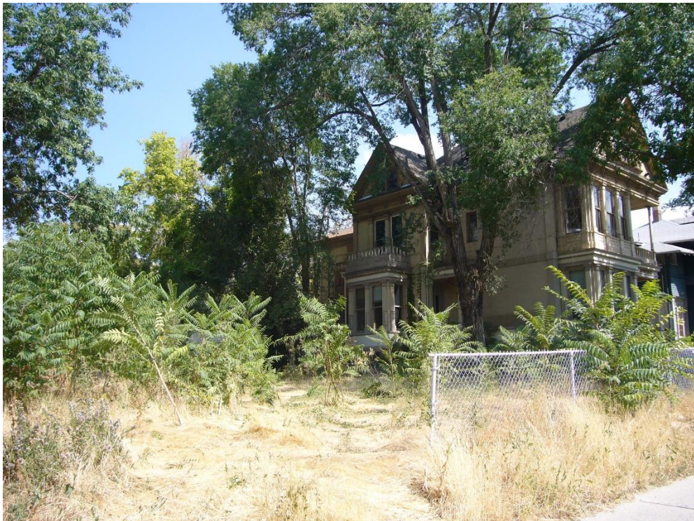
Subject property looking northeast
