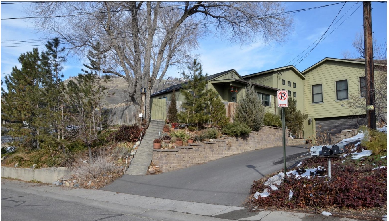
WEST CAPITOL STREET – EAST SIDE
