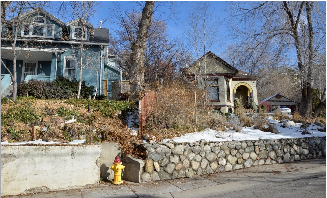
WEST CAPITOL STREET – EAST SIDE (MOVING SOUTH)
