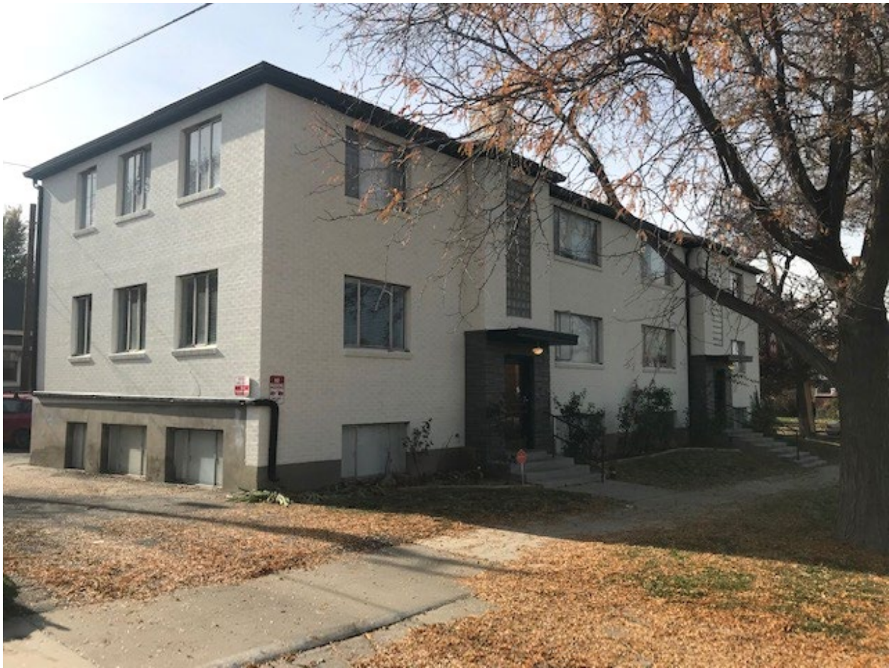
Image 3 – Building after paint was applied
