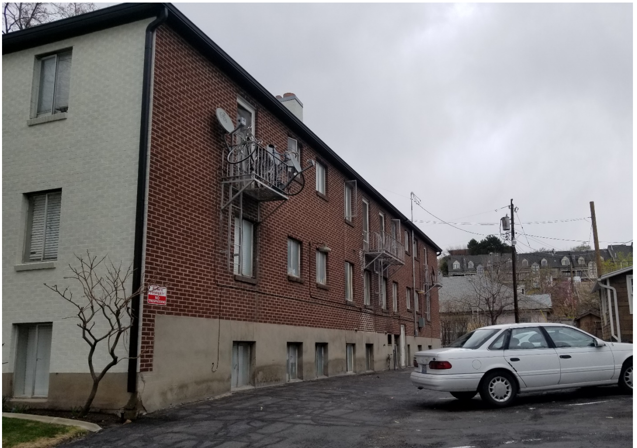
Image 12 – The rear (south) façade was left unpainted
