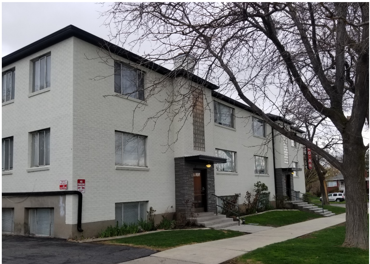
Image 10 – Closer view of the east and north facades of the building after paint was applied
