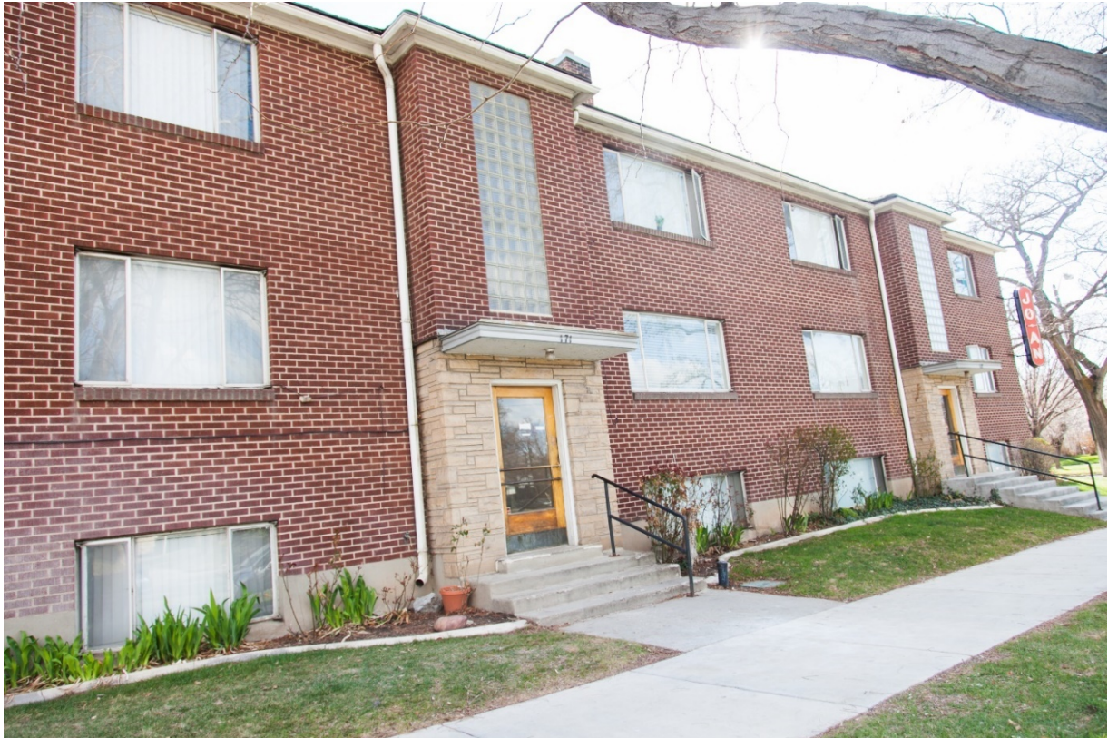
Image 1 – Front (north) façade of the apartment building before paint work was completed.
