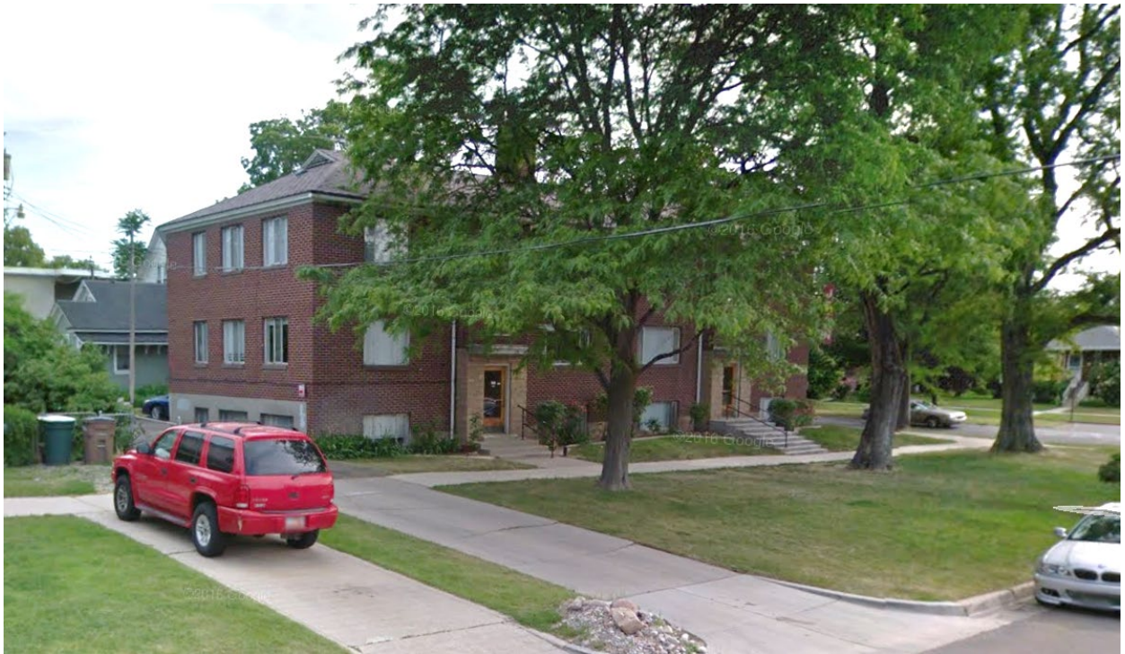
Image 7 - Google street view from June 2016 shows the unpainted east and north façades of the building
