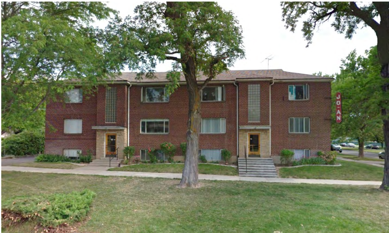
Image 6 – Google street view from June 2016 shows the unpainted front (north) façade of the building
