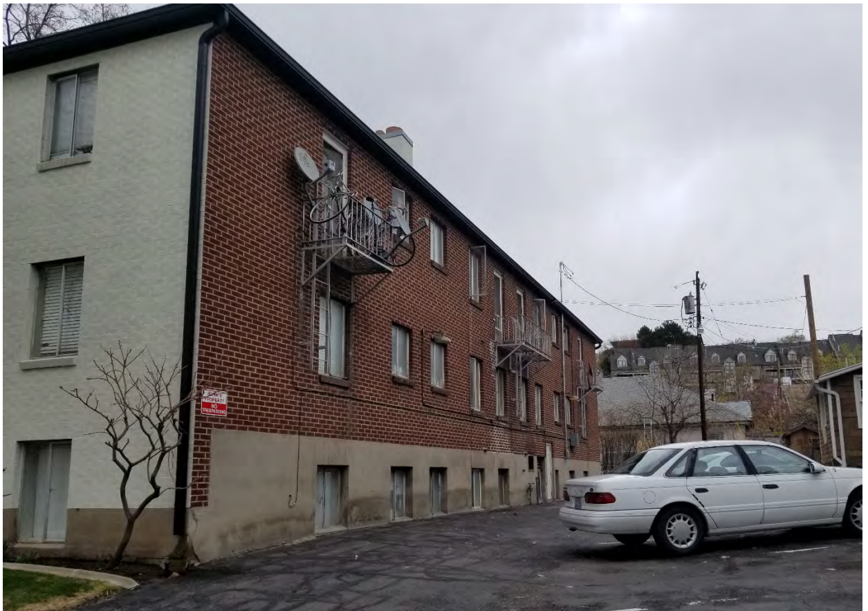
Image 12 – The rear (south) façade was left unpainted
