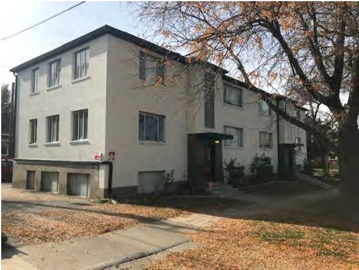
Image 3 – Building after paint was applied
