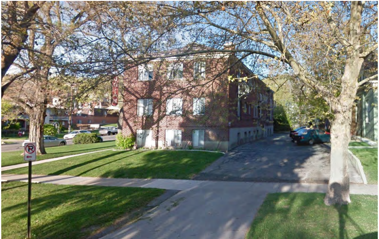
Image 8 - Google street view from June 2016 shows the unpainted west and south façades of the building
