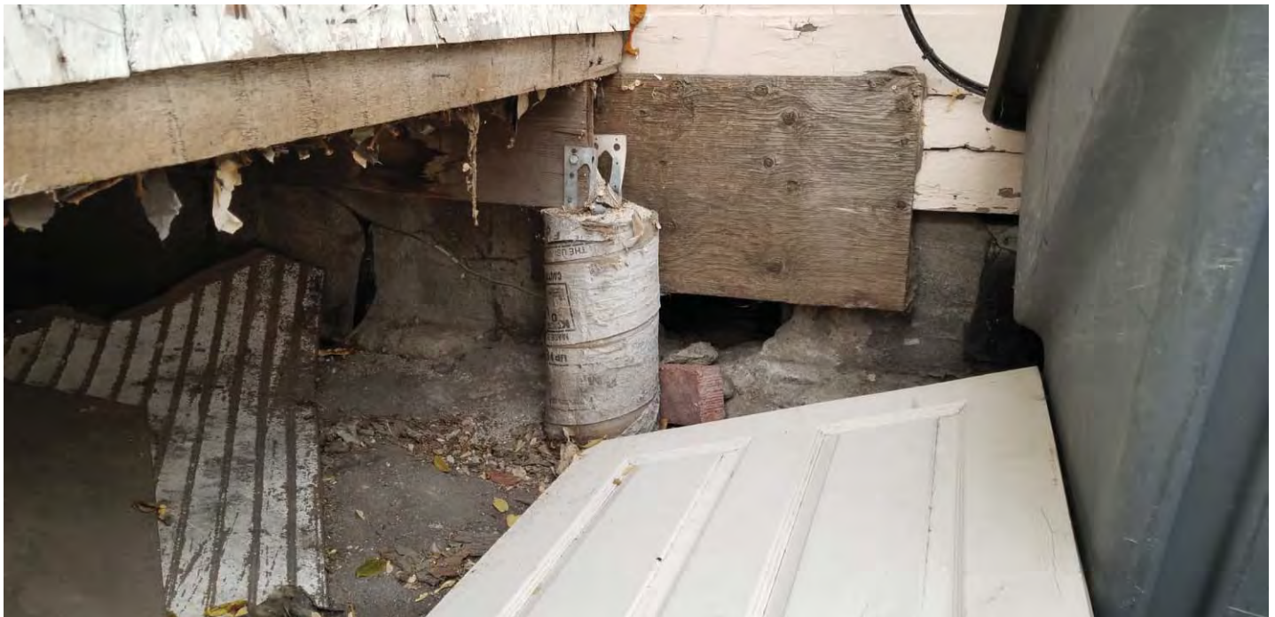
PHOTO #24 PHOTO OF BUILDING #4 AND THE FOUNDATION DAMAGE AND DETERIORATED BEAM FOR THE BACK ROOM.
