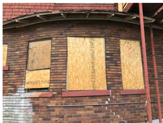
Image 06 - Significant settlement and large cracks in the brick veneer
