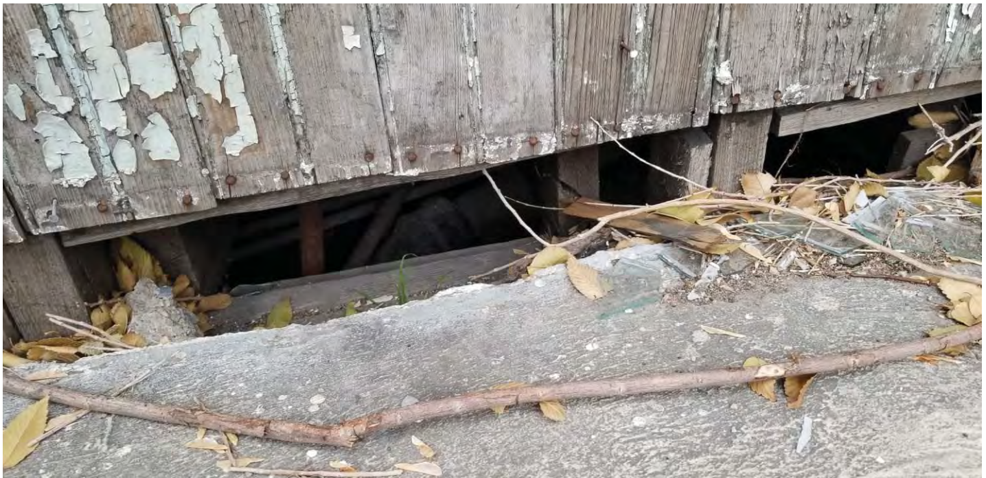
PHOTO #8 PHOTO OF CONCRETE SLAB/CURB AND SOME CRACKING/DETERIORATION OF JOISTS AT THE WALL AT BUILDING #2.
