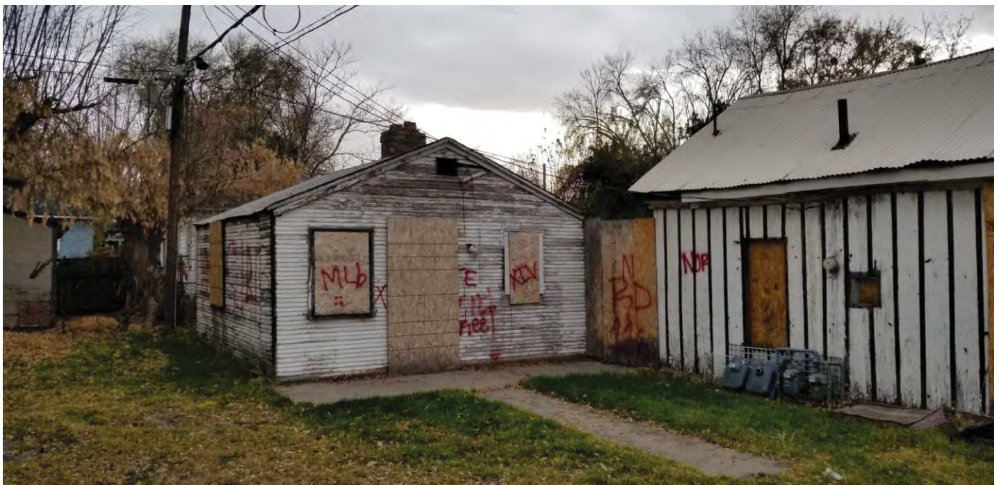
PHOTO #28 PHOTO OF BUILDING #5. SAGGING ROOFS ARE VISIBLE IN THIS PHOTO.
