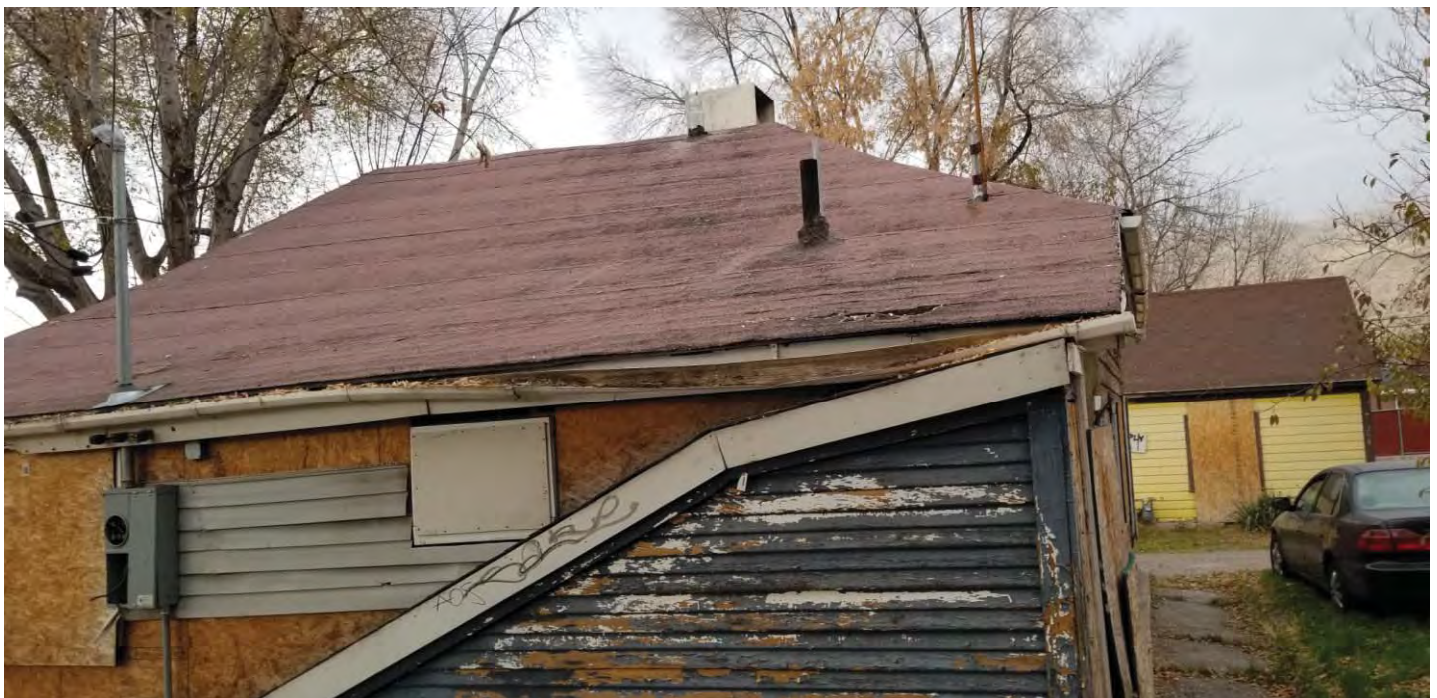
PHOTO #54 PHOTO OF BUILDING #8. THE ROOF HAD SOME VISIBLE DEFLECTIONS.
