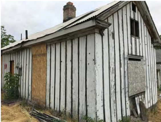
Image 01 - Rotting wood structure
