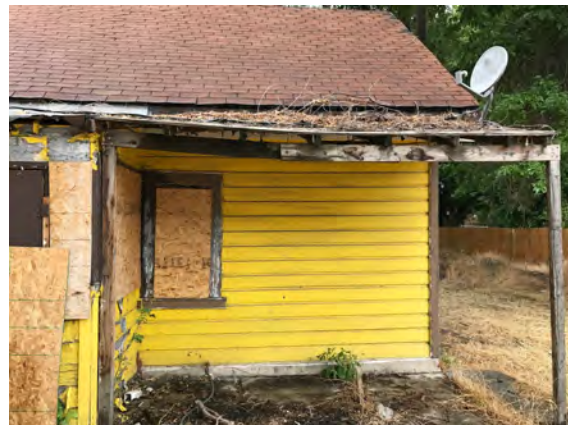
Image 04 - Rotting wood structure with roof on the verge of collapse
