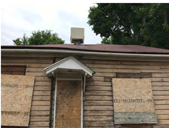
Image 05 - Rotting wood structure and significant sag in the roof.
