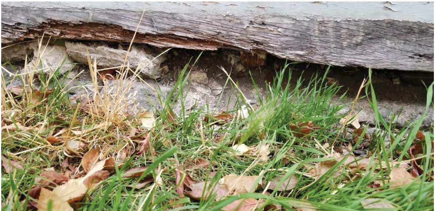
PHOTO #42 PHOTO OF DETERIORATING WOOD AT THE BASE OF BUILDING #7.
