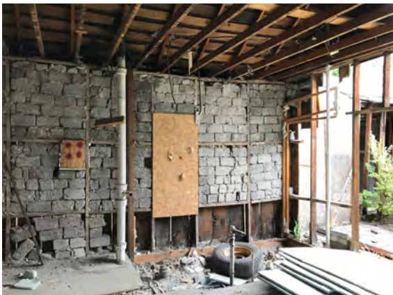
Image 03 - Interior of wood framed with rotting wood and unstable. Not safe to occupy.
