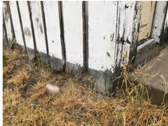
Image 02 - No adequate foundation support
