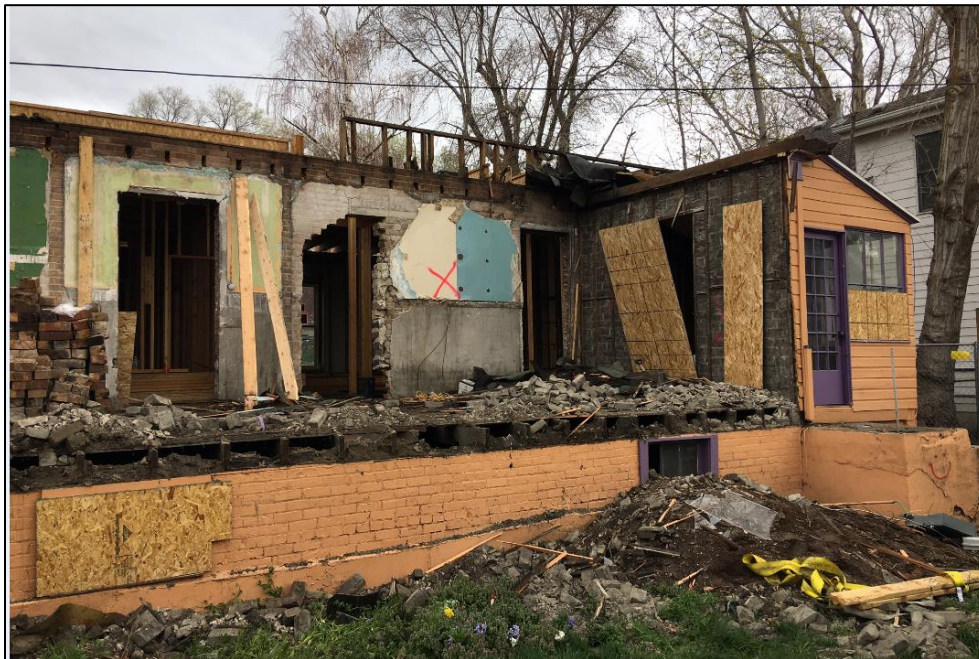
Photo of Subject Property Post Collapse.
