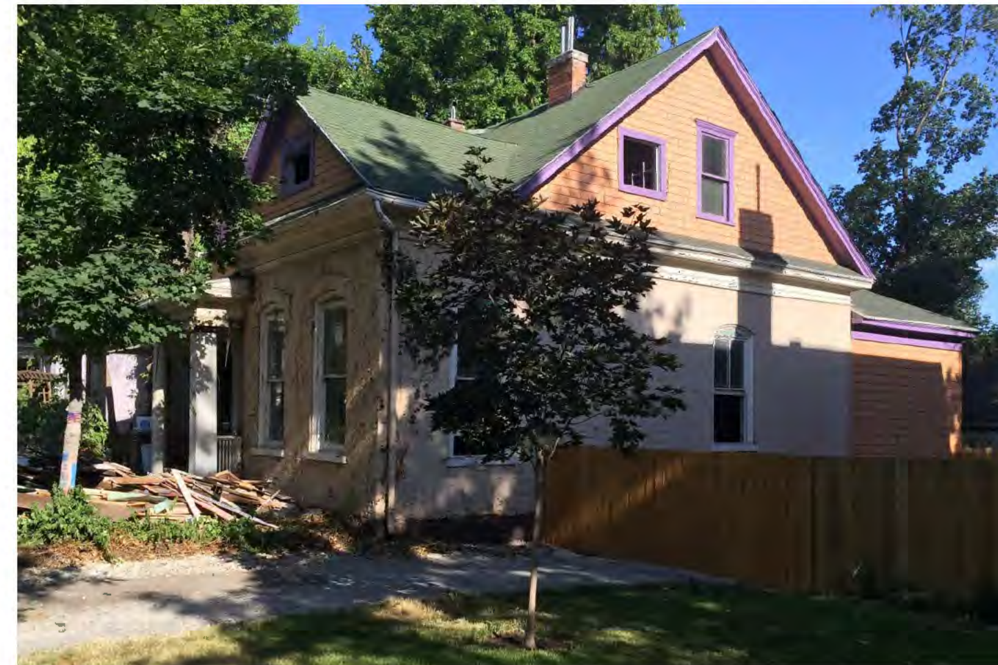
EXISTING NORTH WEST VIEW [ PRIOR TO 2017 EVENT ]
