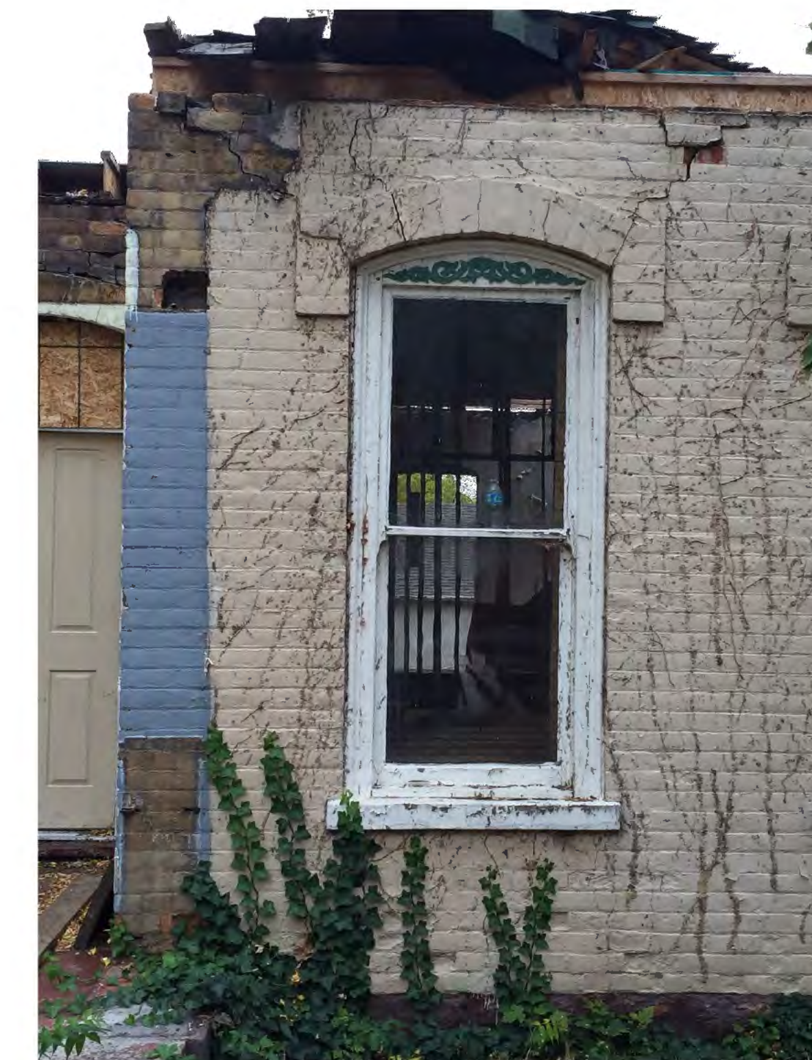
772 E 2nd AVENUE - CURRENT CONDITIONS - NORTH-WEST WINDOW
