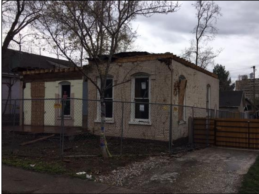
Photo of Subject Property Post Collapse.
