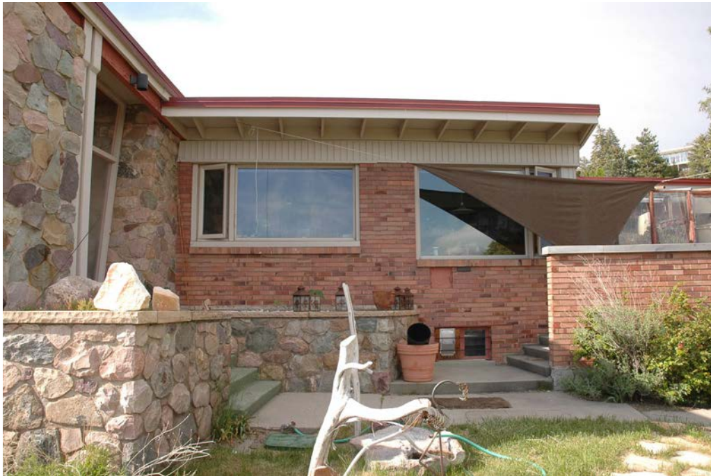
Photograph 3 South elevation of house, east half. Camera facing north.
