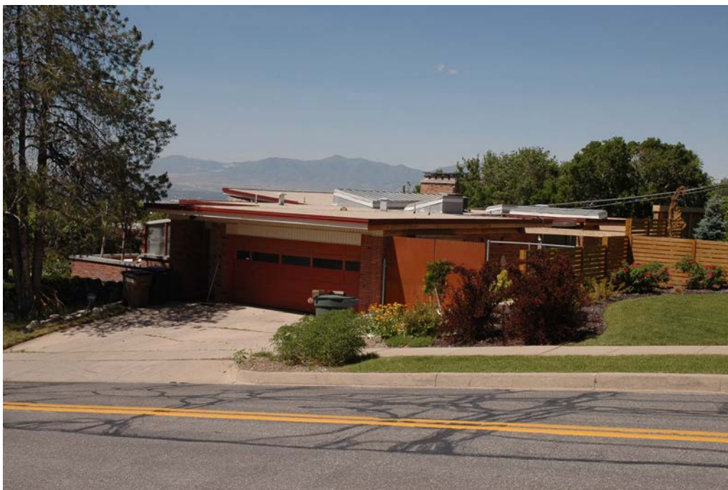
Photograph 2 East and north elevations of house. Camera facing southwest.
