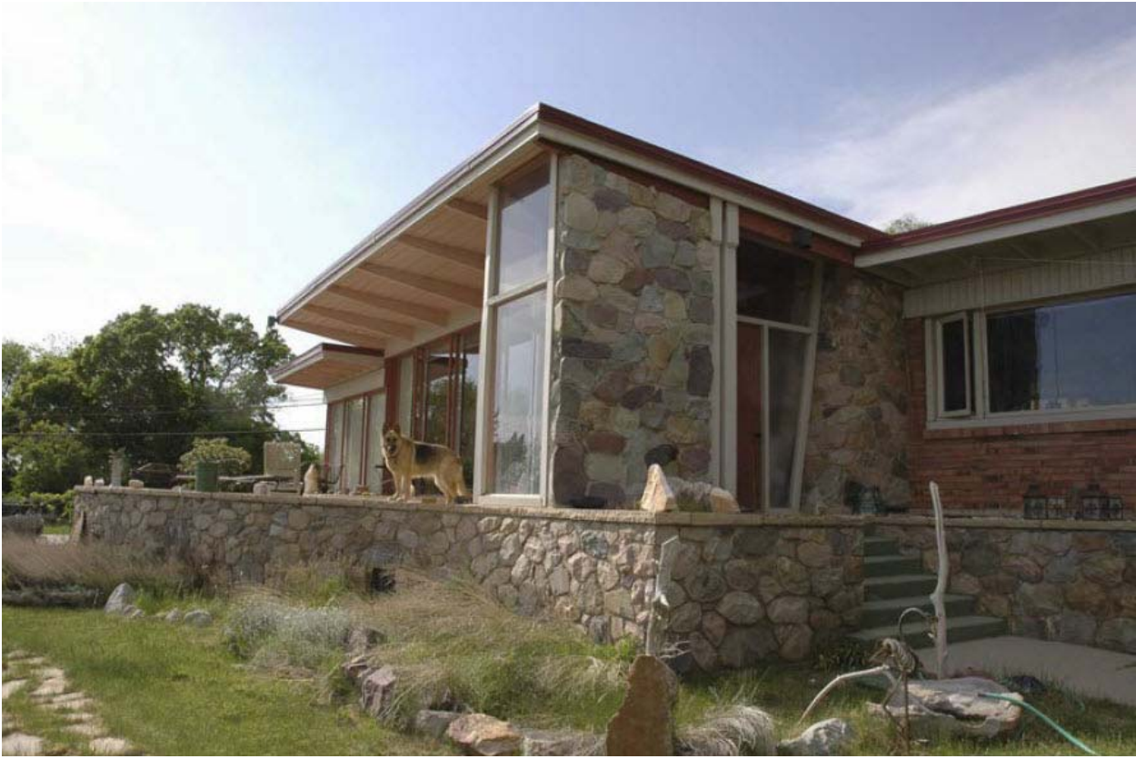
South and east elevations, 2017
