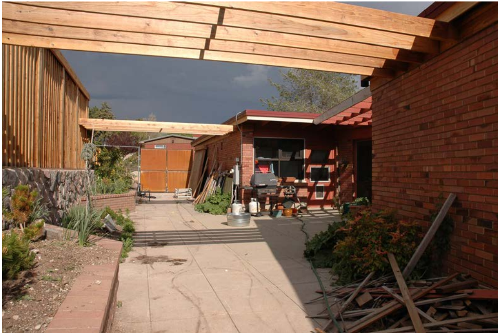
Photograph 7 North elevation of house. Camera facing east.
