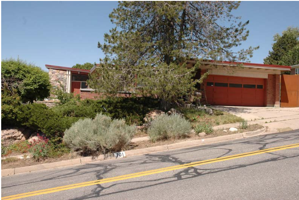
Photograph 1 East elevation of house. Camera facing west.
