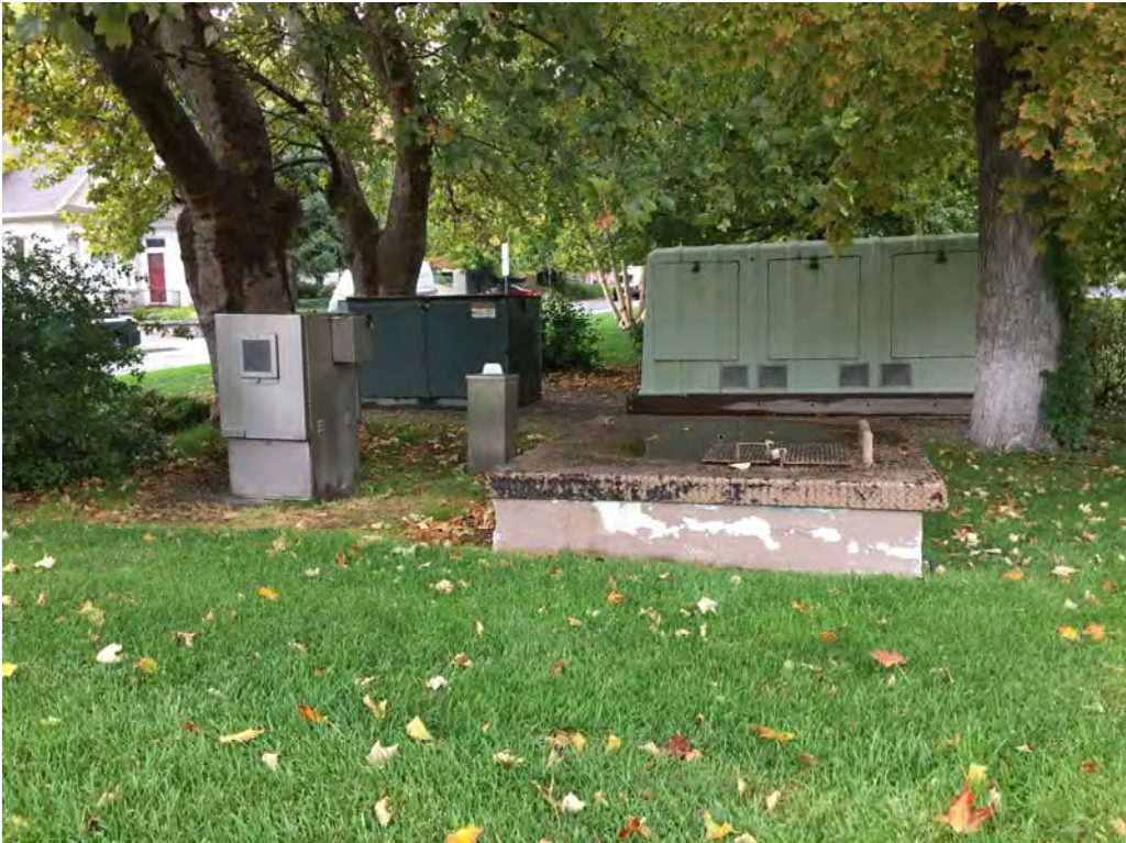
Photo #2: Existing Well Looking North
