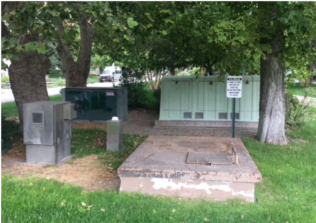
View of Existing Well
