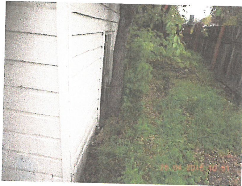
Photo 13 – Retained soils at the north exterior wall
