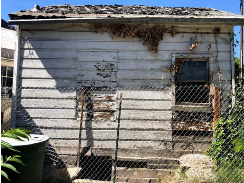
Image 3- Existing South exterior wall (to be restored)
