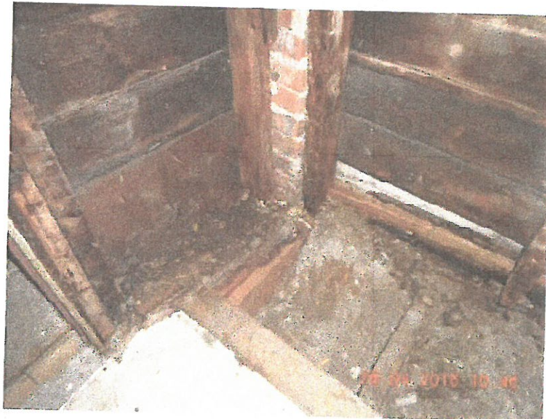
Photo 8 – Masonry infill in wall cavity
