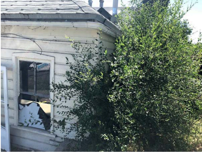
Image 5- Existing North exterior wall (to be restored)
