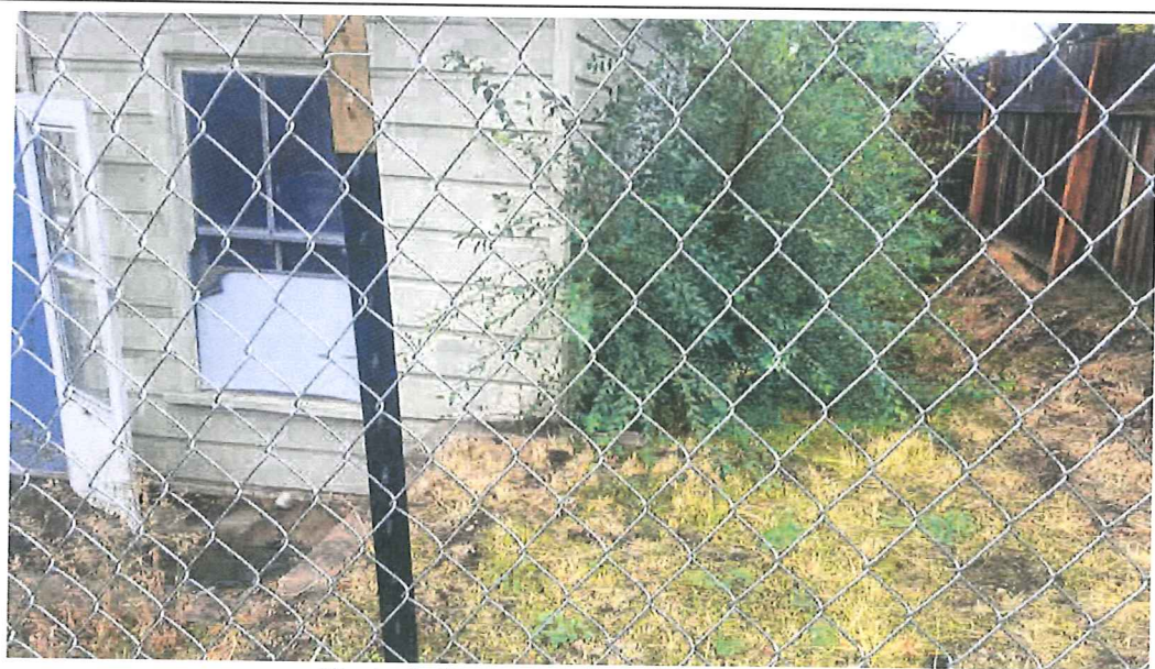
Photo 4: Home constructed below grade.
