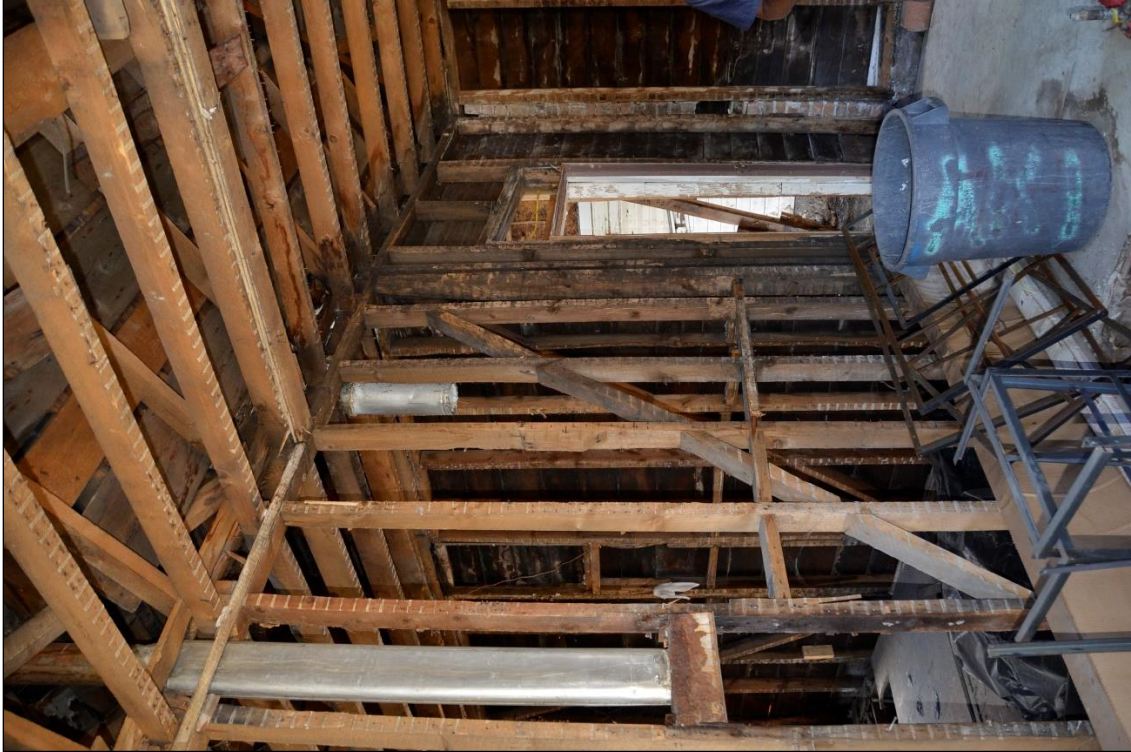
Looking South West
