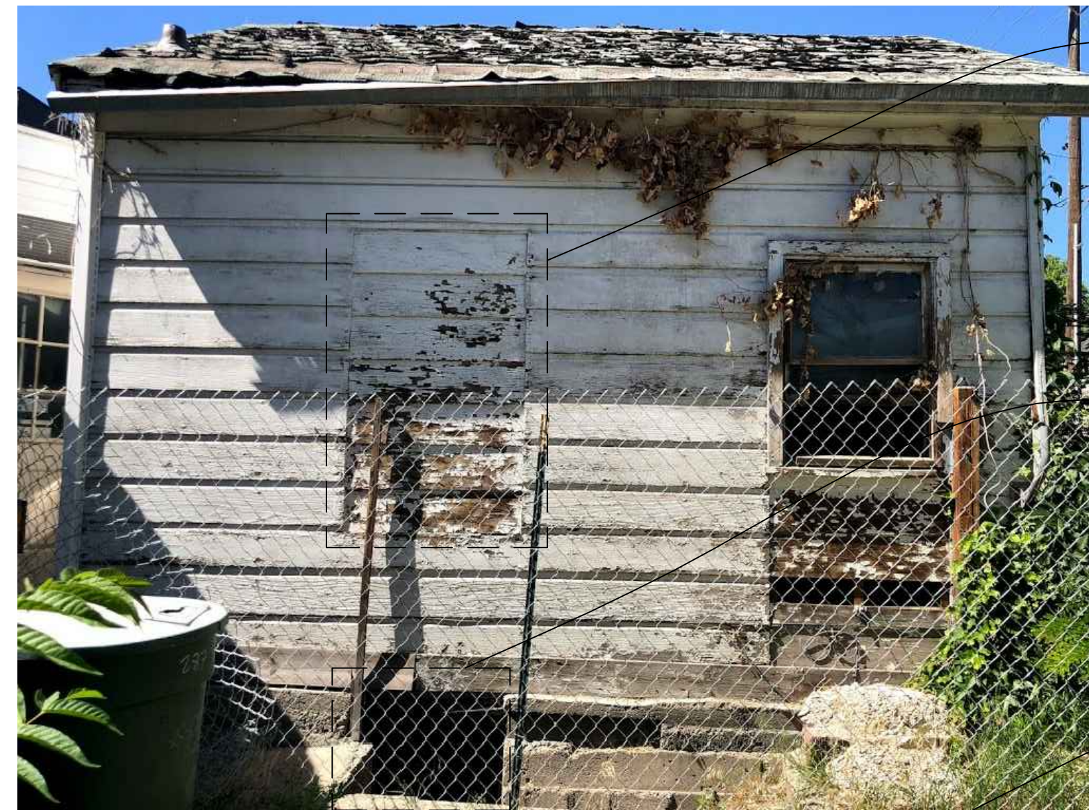
PHOTOGRAPHY OF THE SOUTH WALL OF THE HOUSE
