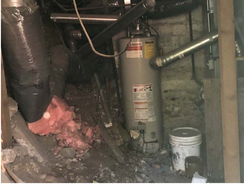
Image 7 - Existing basement/foundation (to be replaced.)
