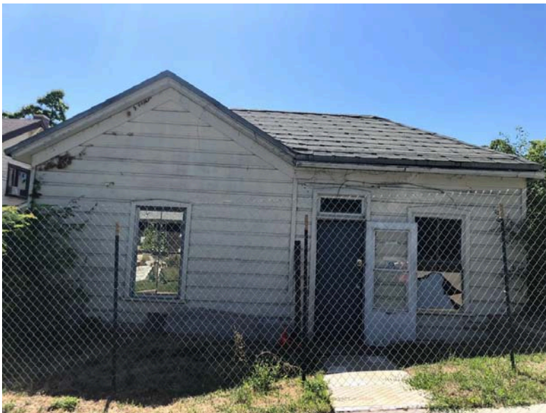
Image 4- Existing East exterior wall (to be restored)
