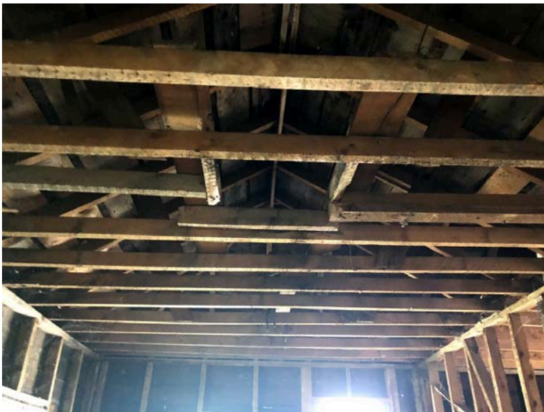
Image 6 - Existing roof ( to be reinforced and restored)
