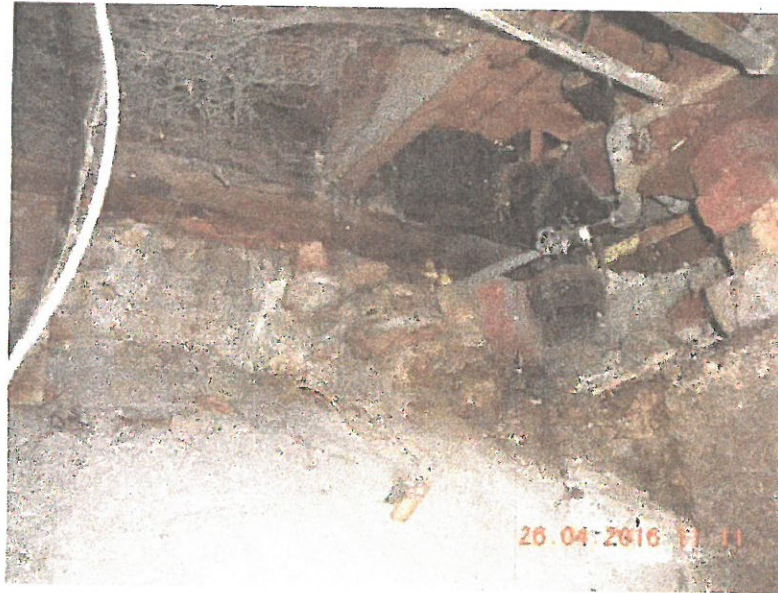
Photo 5 – Inadequate load transfer connection at deteriorating foundation
