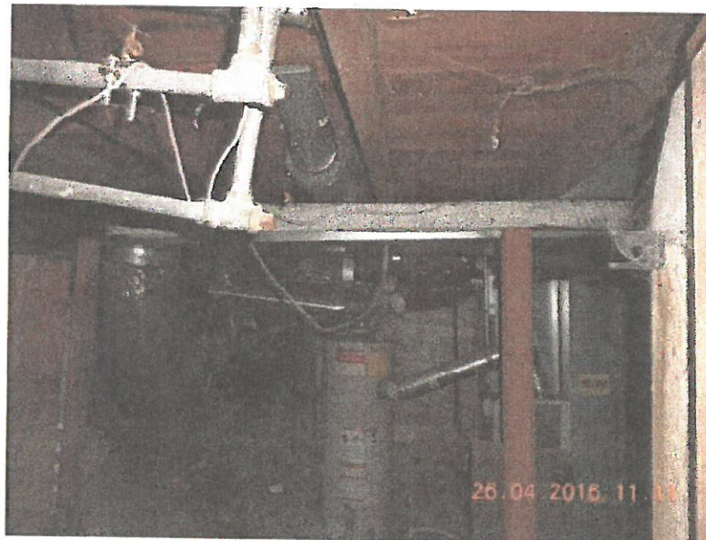
Photo 6 – Apparent added shoring for floor support
