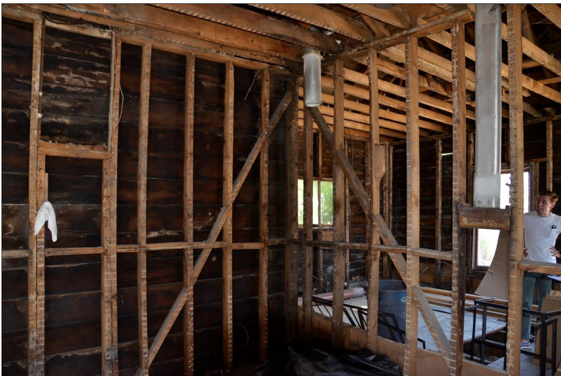
Looking NW from South Wing
