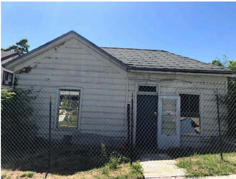
Image 4- Existing East exterior wall (to be restored)
