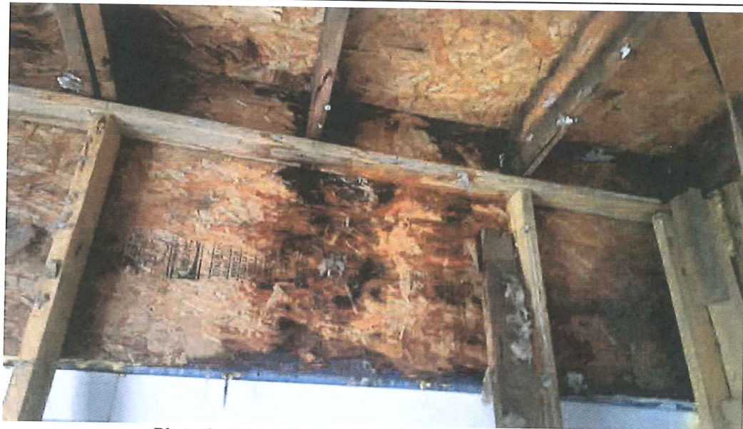
Photo 2: Water damage from improper roof drainage
