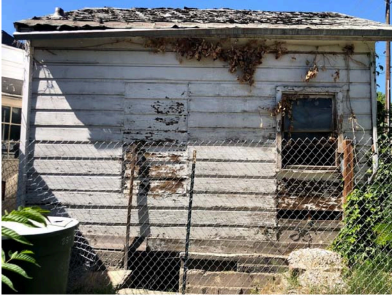
Image 3- Existing South exterior wall (to be restored)
