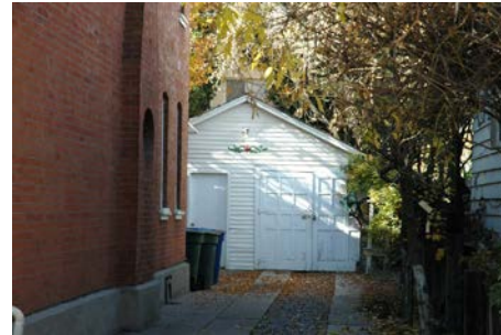
229 “C” Street (garage)
