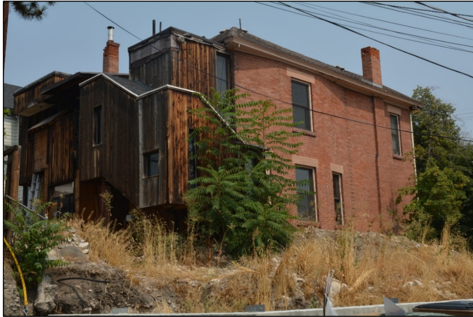
Southwest perspective of historic home and existing addition
