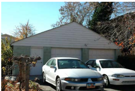
237 “C” Street (garage)
