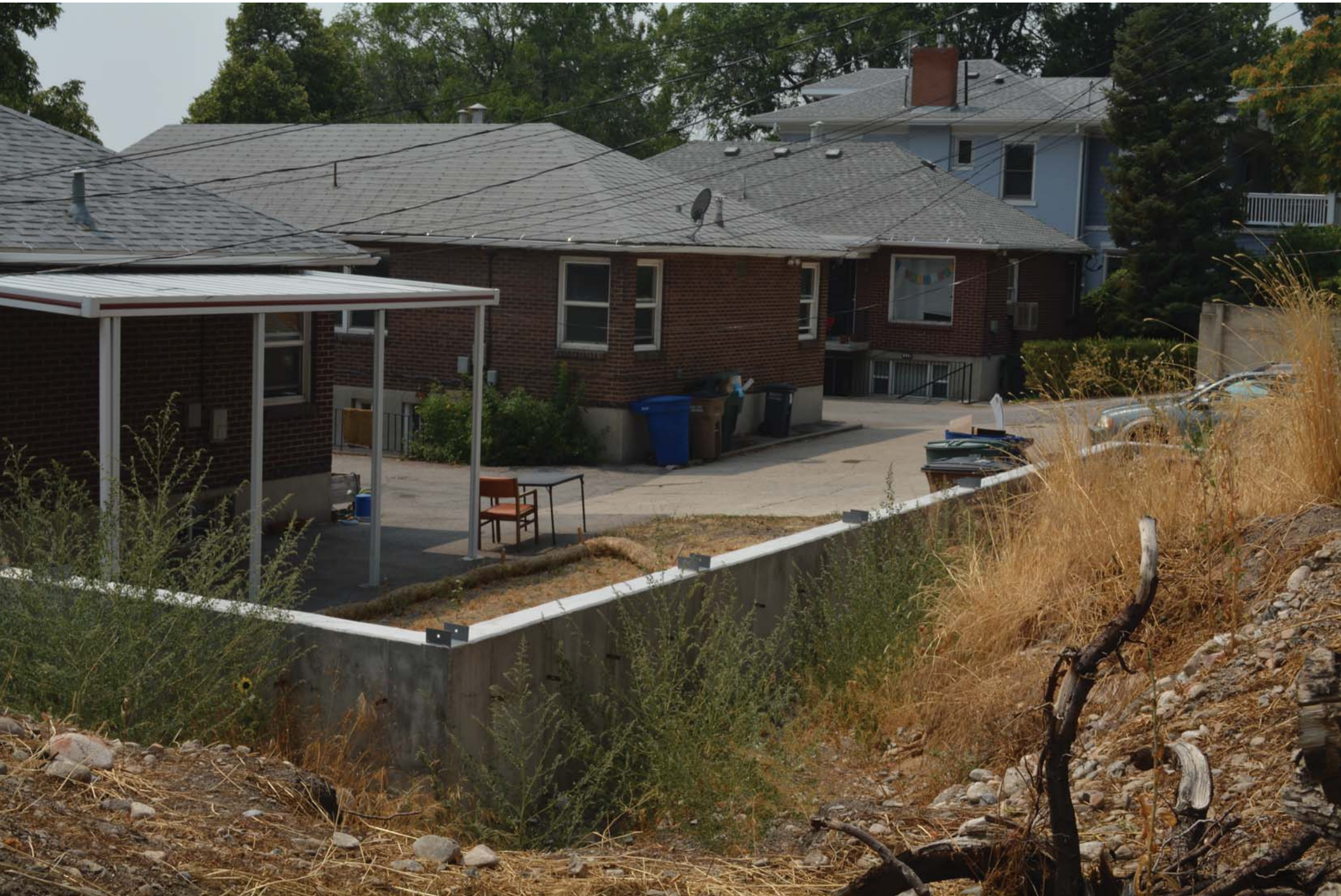
Retaining wall that runs along southwest property line of site
