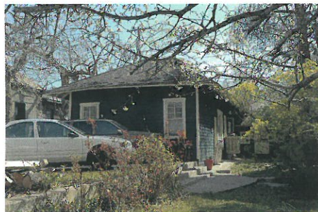
1007 E 1 st Avenue (garage)
