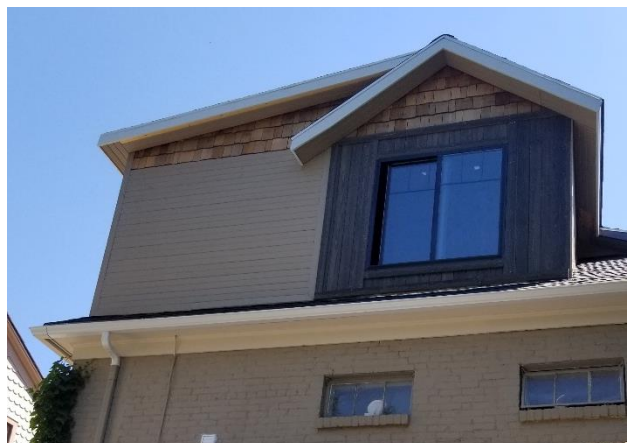
Figure 5 – Cladding of rooftop addition includes wood shingles, pine siding and rough sawn shiplap panels.
