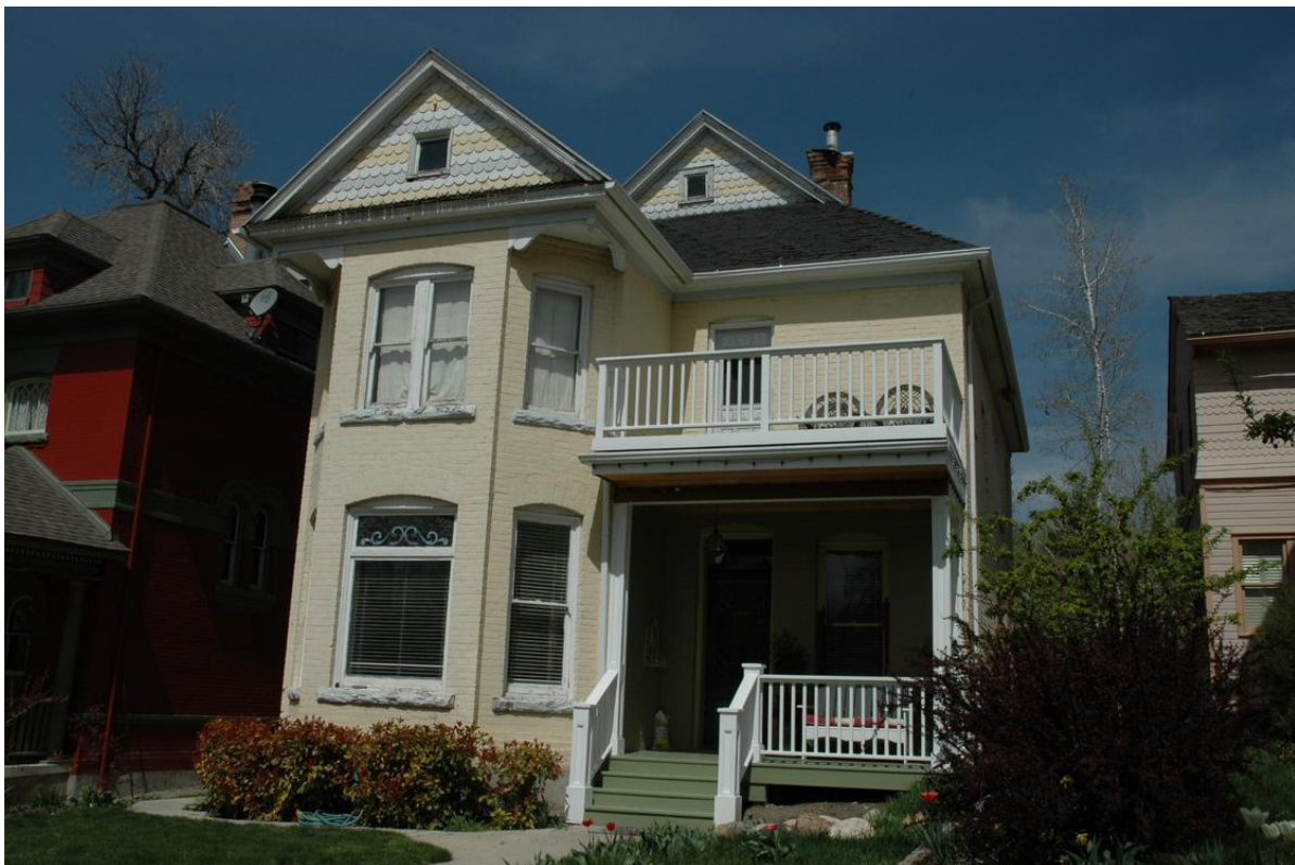
Figure 6 – Front façade of the historic home in 2007.
