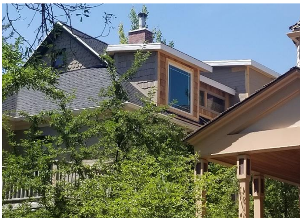
Figure 4 – Dormers were cladded with wood shingles
