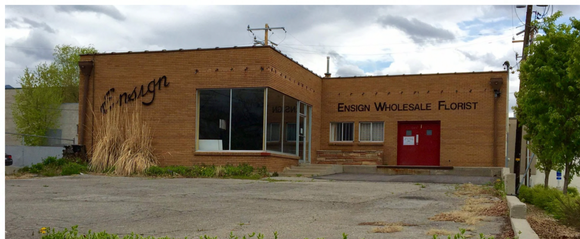
EXISTING WEST FACADE
