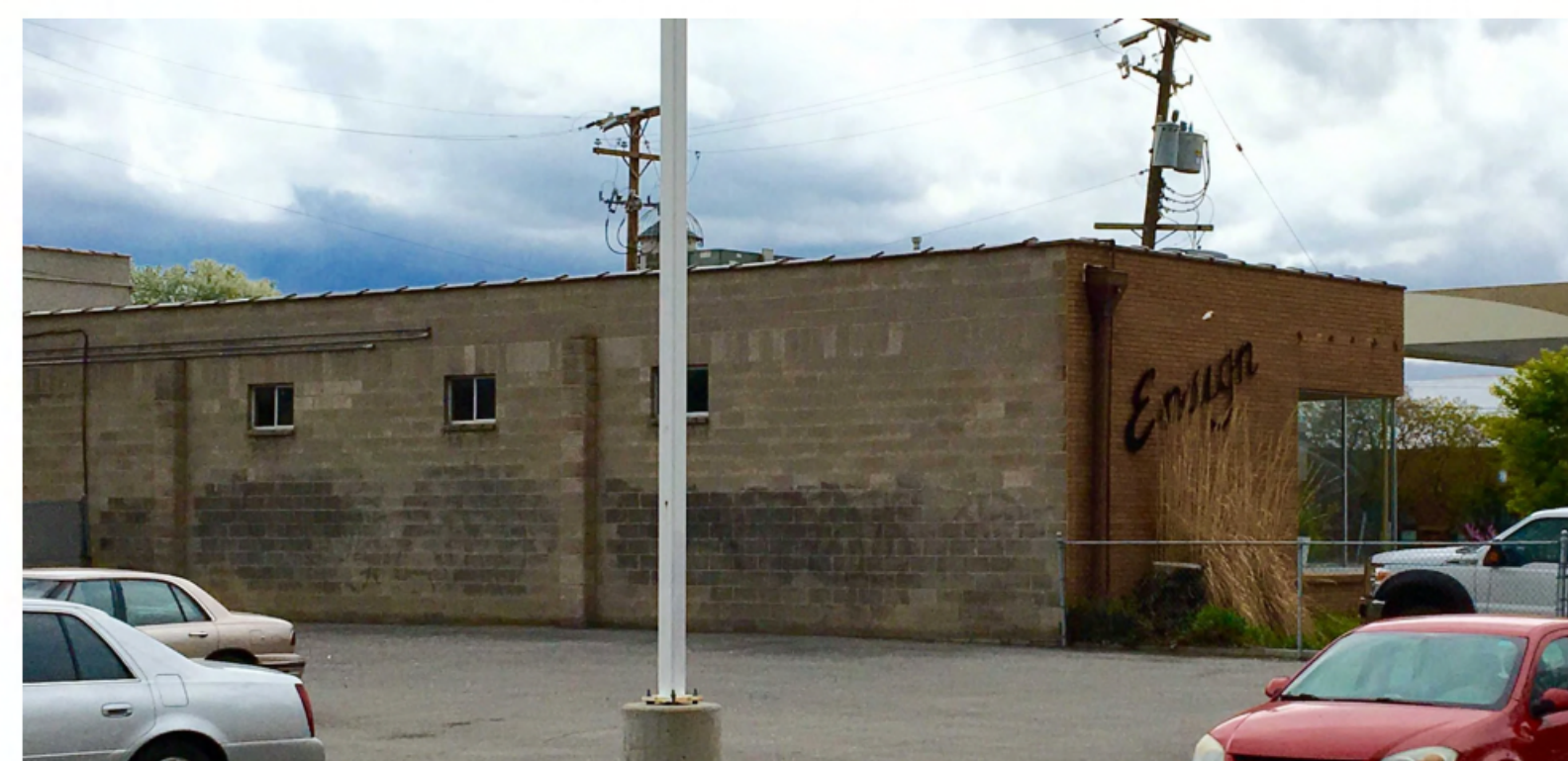
EXISTING NORTH FACADE
