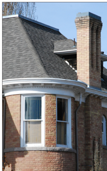
Asphalt shingles are the typical and appropriate roofing material for this style and period of architecture.
