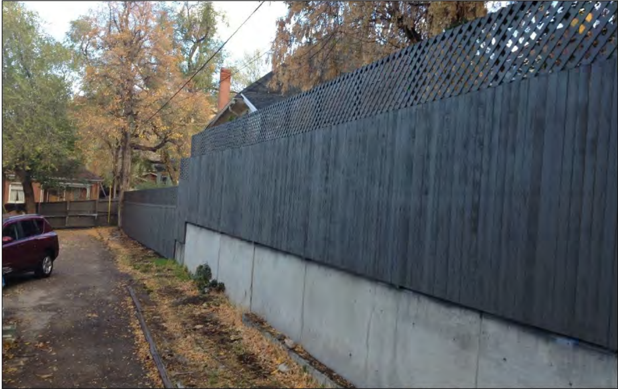
Northward View of Finished Fence in Rear Yard of Subject Property
