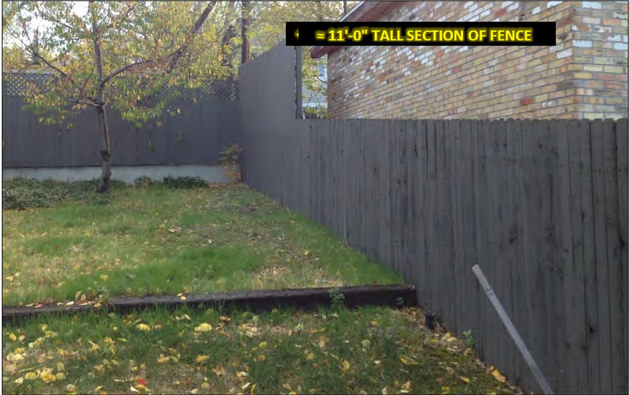
Intersection of Interior Side Yard & Rear Yard Fence Line at Southeast Corner of Lot
