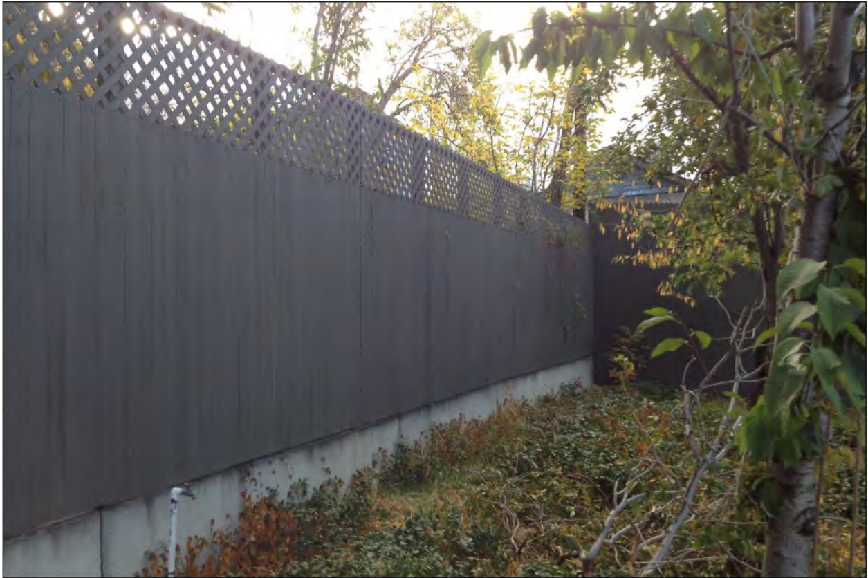
Intersection of Rear Yard Fence & Side Yard Fence at Southeast Corner of Lot
