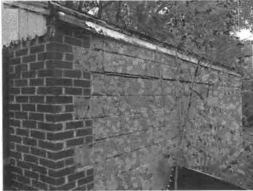
Out-of-plumb block walls at garage structure
