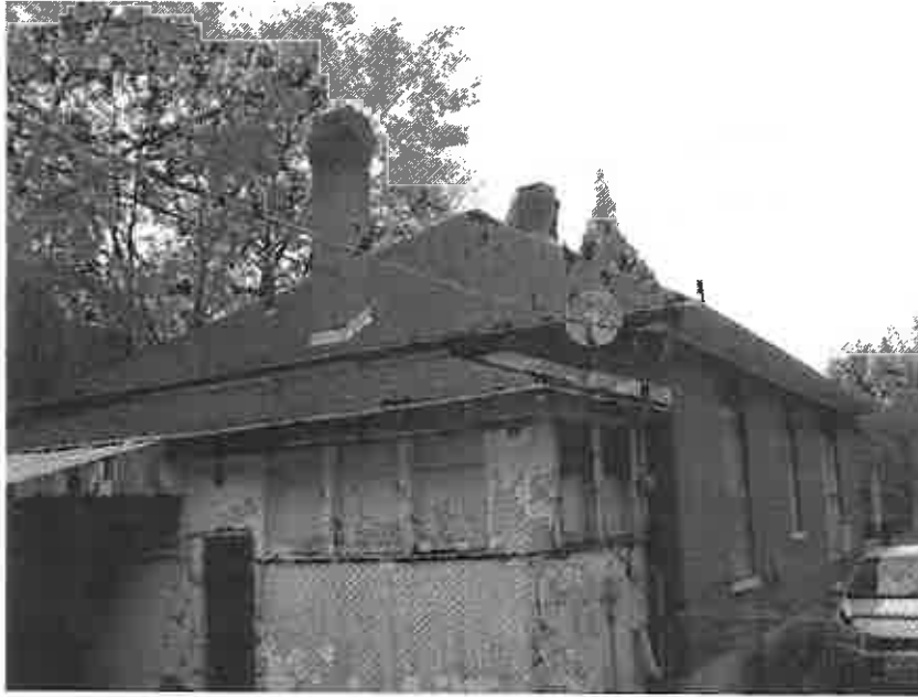
Chimney requires bracing and the roof is sagging behind the chimney
