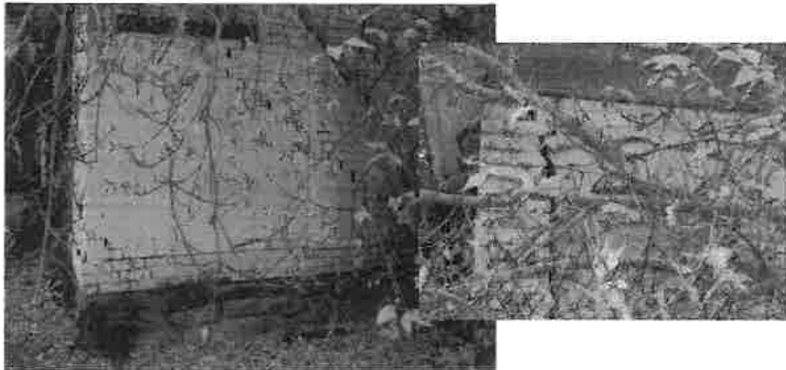
Foundation settlement in North-West corner has caused walls to crack and separate
