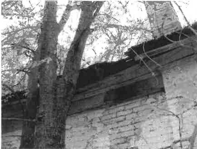
Trees have damaged the roof structure and have allowed water to enter the attic and wall cavities
