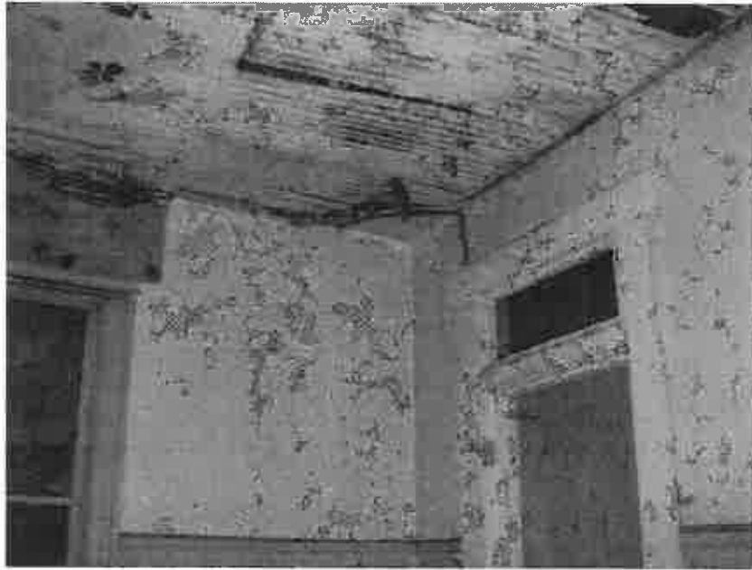
The roof is damaged and has allowed moisture to rot out the ceiling and attic floor
