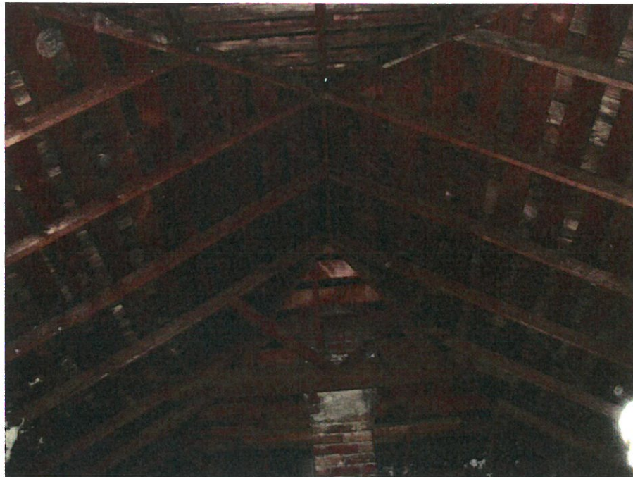
Roof framing and un-reinforced brick chimney
