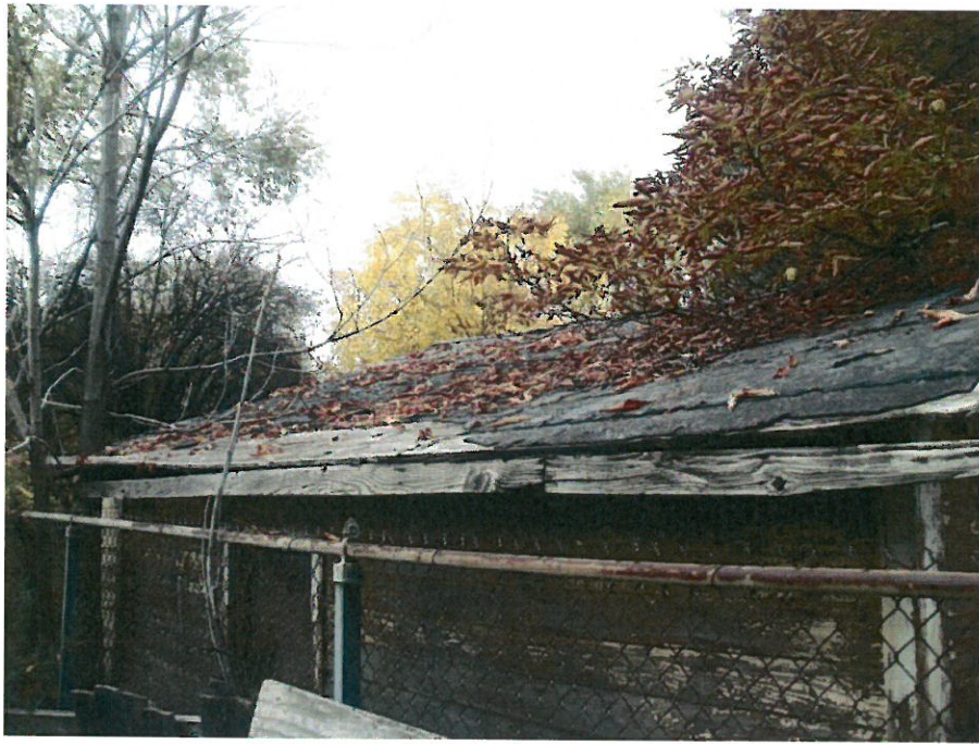
The roof for the shed is sagging and severely deteriorated
