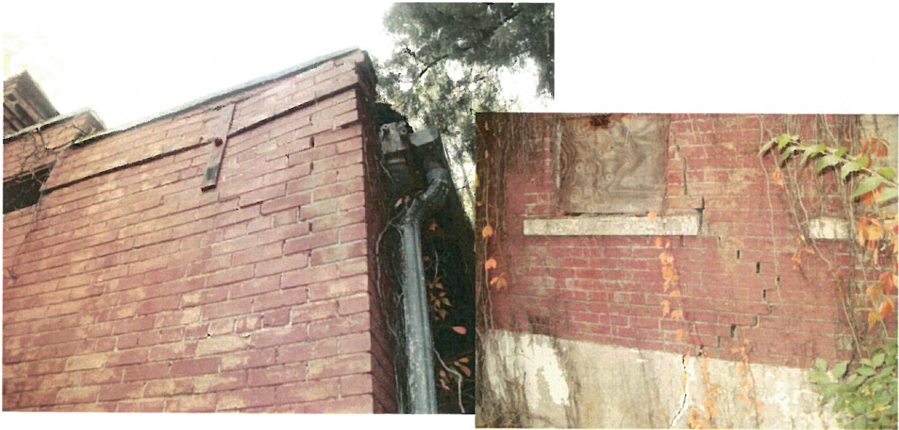
Foundation settlement in South-West corner has caused walls to crack and separate
