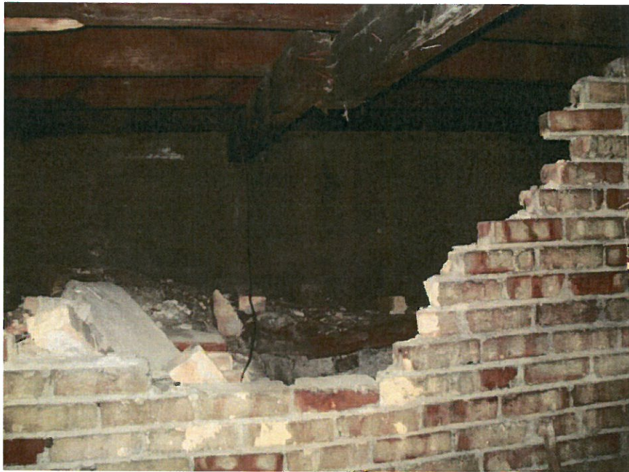
Walls supporting beams in the floor have been damaged, leaving floor joists above unsupported
