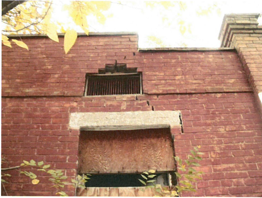
Foundation settlement in South-West corner has caused walls to crack and separate.
